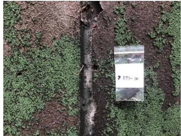
Photo #4 Sample 331-10. Green asphalt rolled sheeting; north shed – not asbestos-containing.
