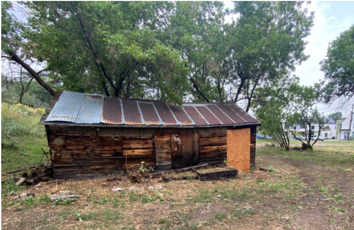
South Side of Shed #1 facing the house at 1302 Norfolk Avenue
