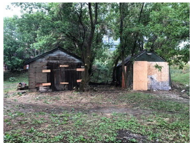
Photo #6 View of east side of both sheds.
