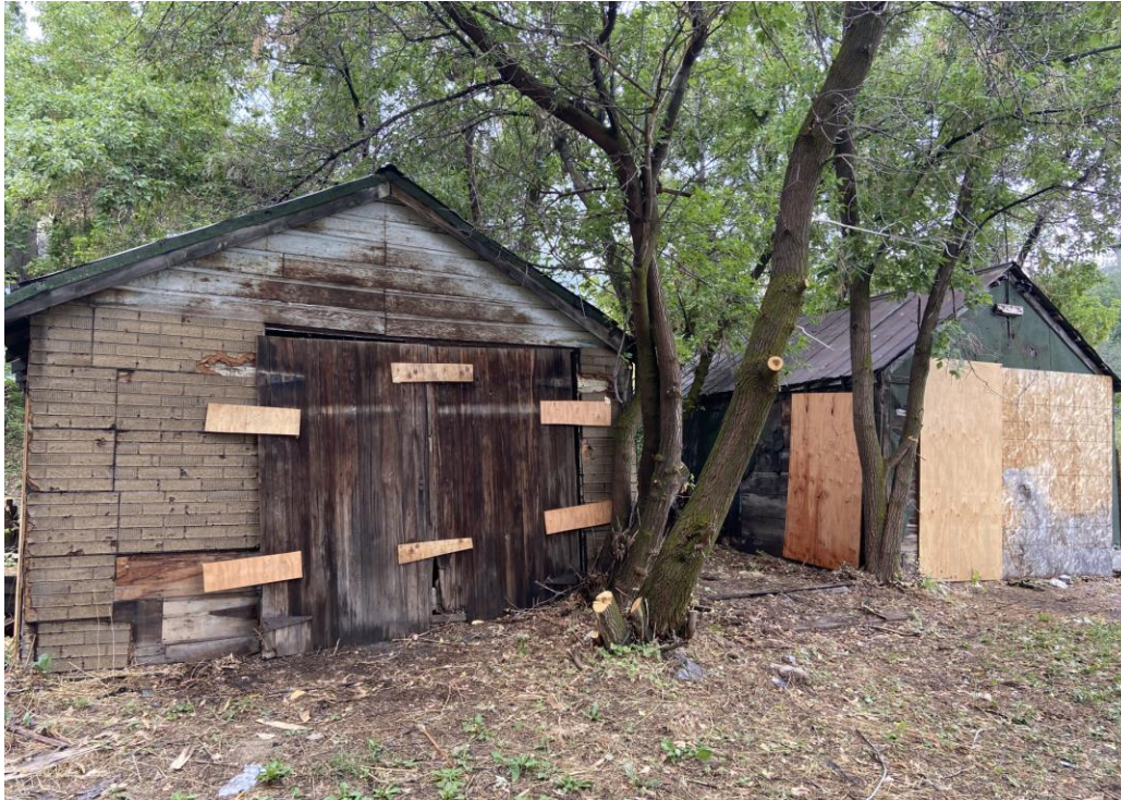
East Side of Shed #1 and Shed #2
