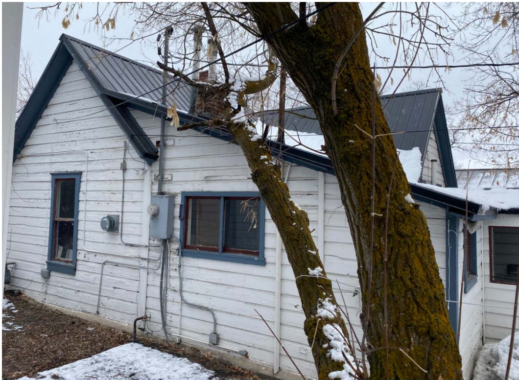
Figure 12: Top; Applicant's Submitted Photograph of South Elevation. Bottom; South Elevation with possible Historic addition in red and non-historic addition in green.
