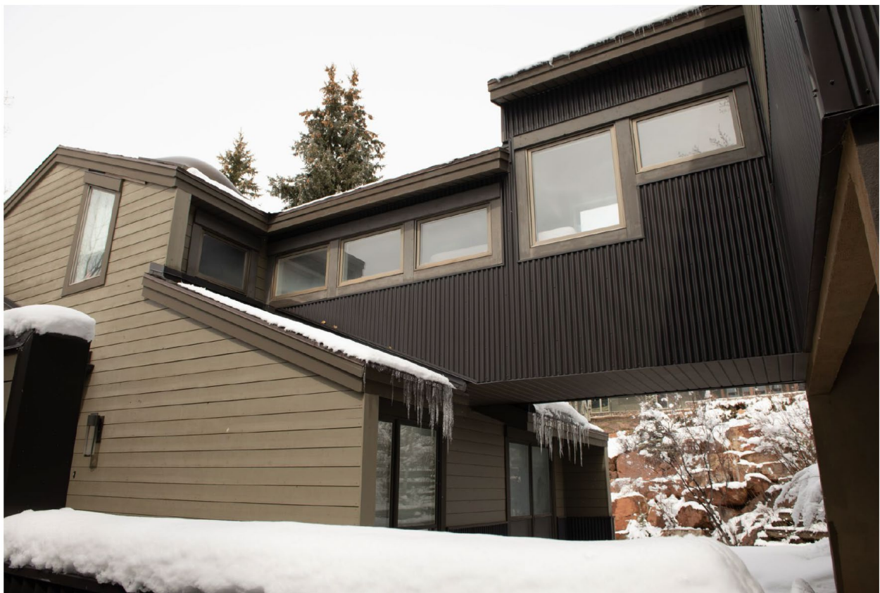
Figure 1 – 2587 Fairway Village Drive elevated walkway
