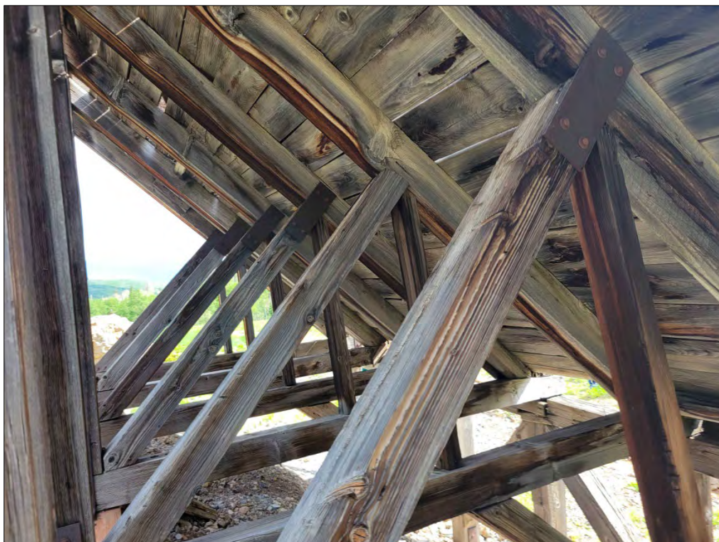
Photo No. 9 Detail of cross brace timbers, sloped floor and mortise-and-tenon joints. Camera facing northwest.
