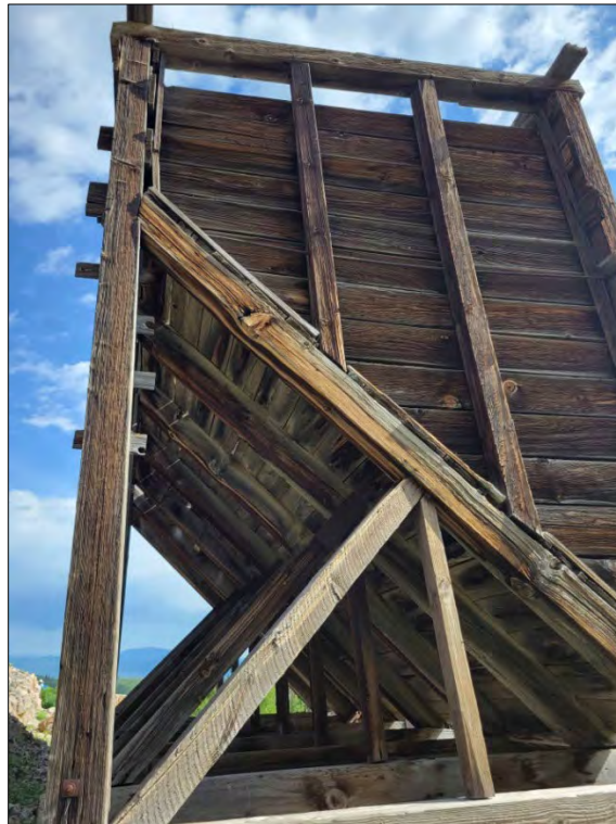
Photo No. 7 South elevation detail showing cross brace timbers. Camera facing north.
