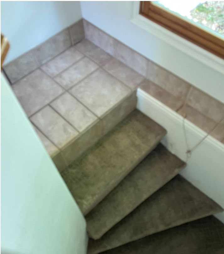
Photo 15.8 – side porch staricase
