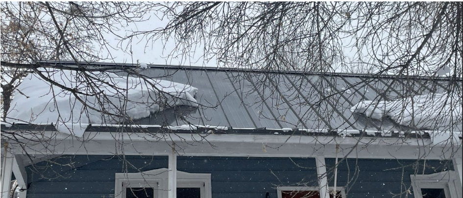
Photo 18.3 – east view roof
