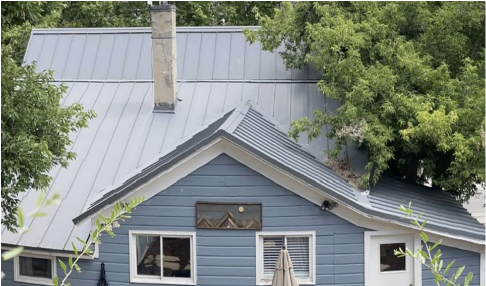
Photo 18.1 – West Elevation Roof
