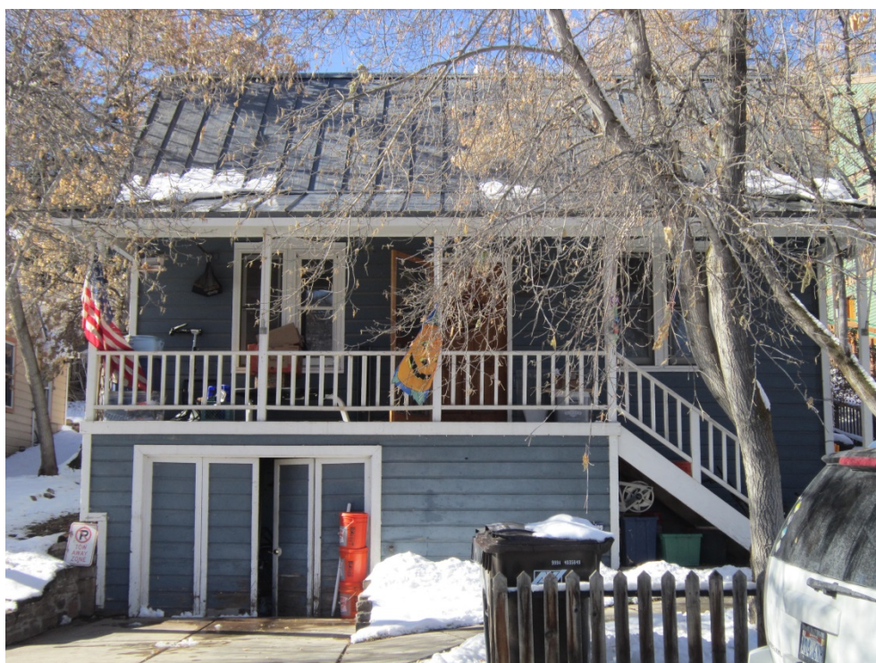
161 Park Avenue. East elevation. November 2013.
