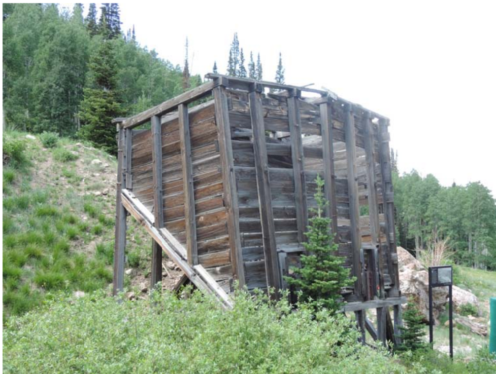
Little Bell Ore Bin. From southeast. June 2016.
