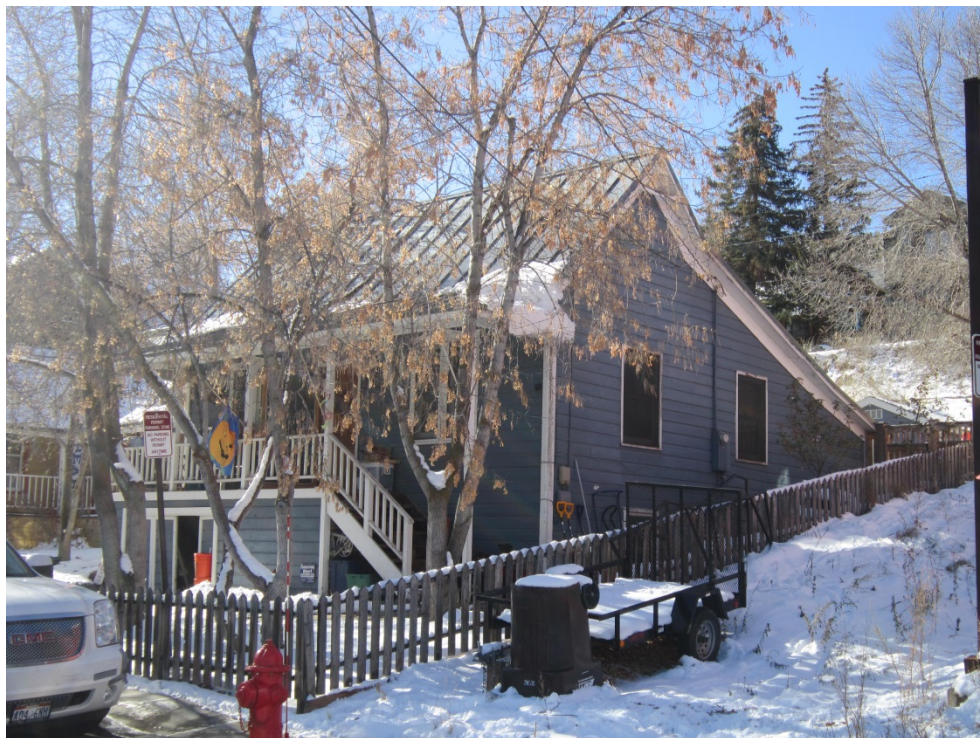
161 Park Avenue. Northeast oblique. November 2013.
