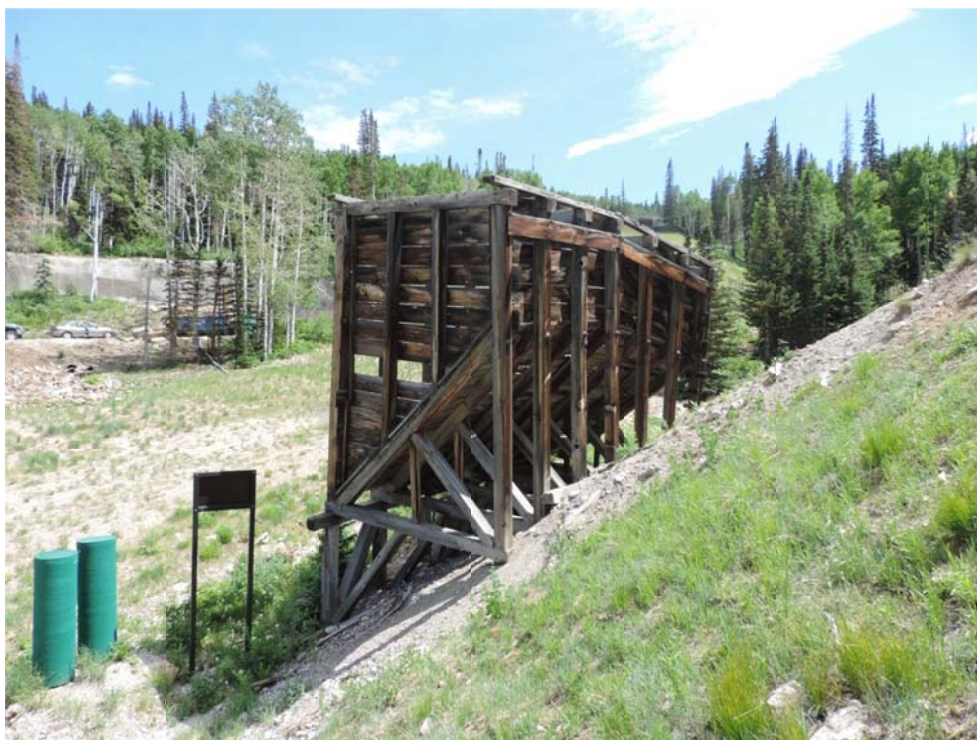
Little Bell Ore Bin. From northwest. June 2016.
