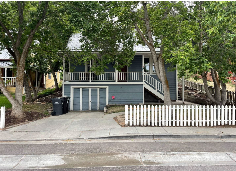
Fig 1. view of property from Park Ave
