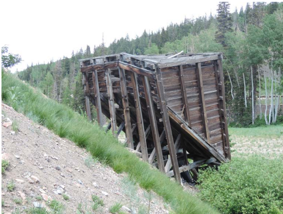
Little Bell Ore Bin. From southwest. June 2016.
