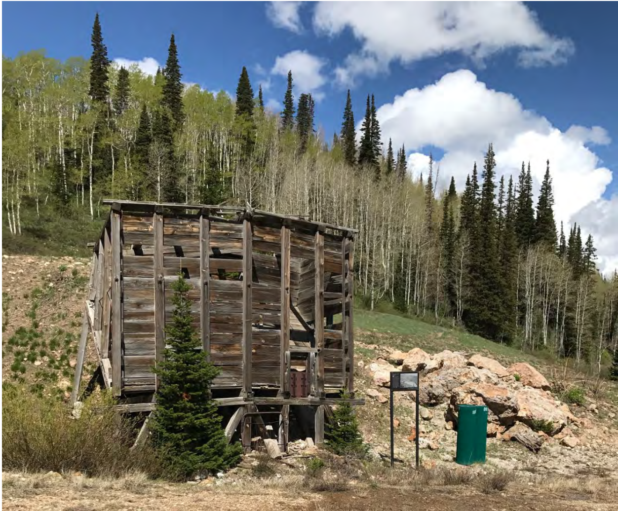
Figure 3. Little Bell ore bin prior to 2017 preservation work. Image courtesy Sandra Morrison.
