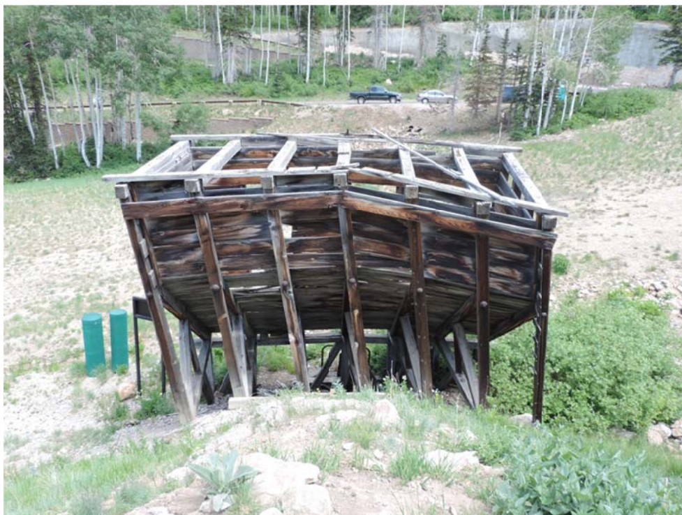
Little Bell Ore Bin. From west. June 2016.
