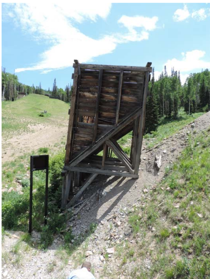
Little Bell Ore Bin. From north. June 2016.
