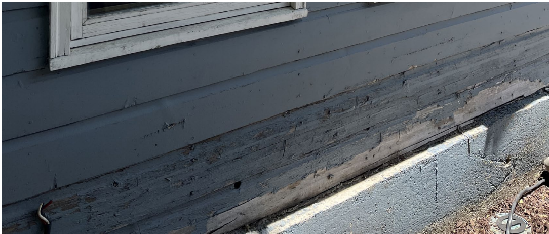
Photo 18.2 – Foundation rear corner
