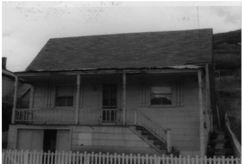
Figure 2: Photo of front facade c. 1945
