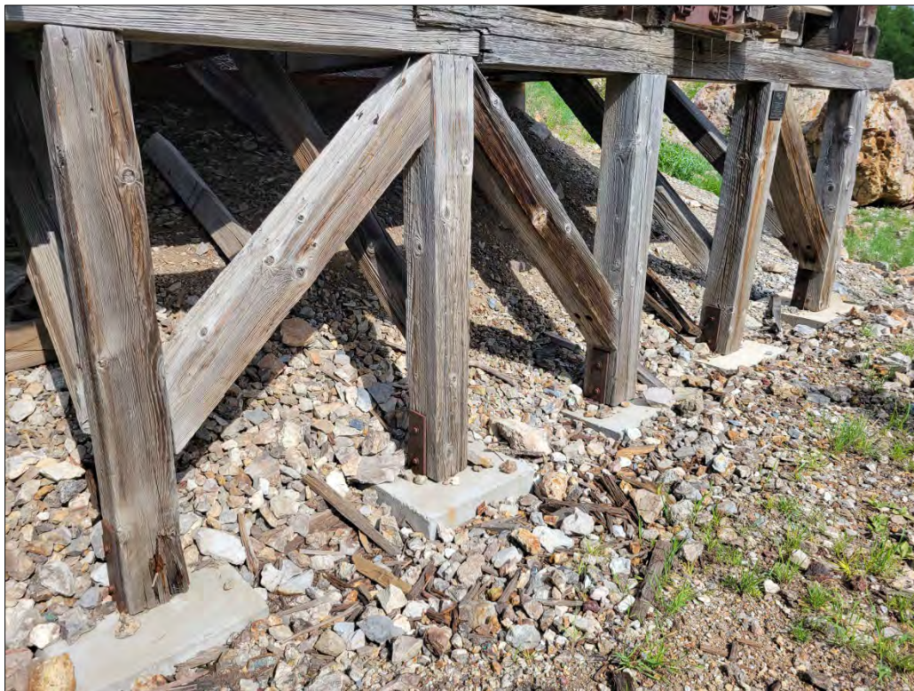
Photo No. 5 Detail of support posts and concrete piers. Camera facing northwest
