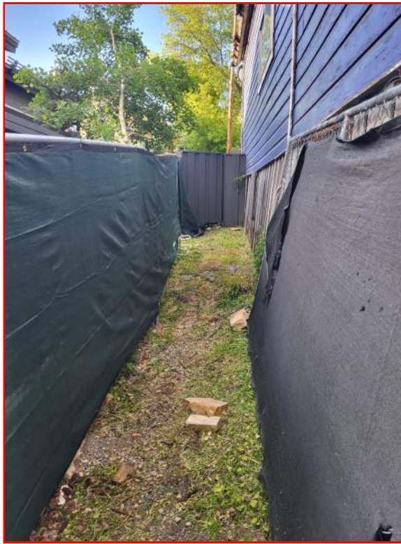
Available Access Along East Side
