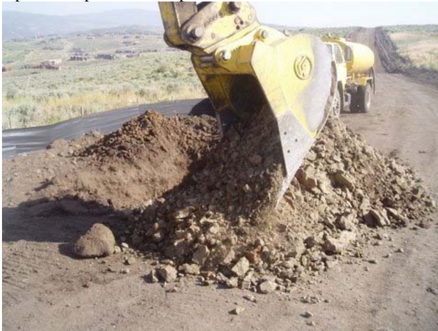
Pipeline test pit excavation pictures.
