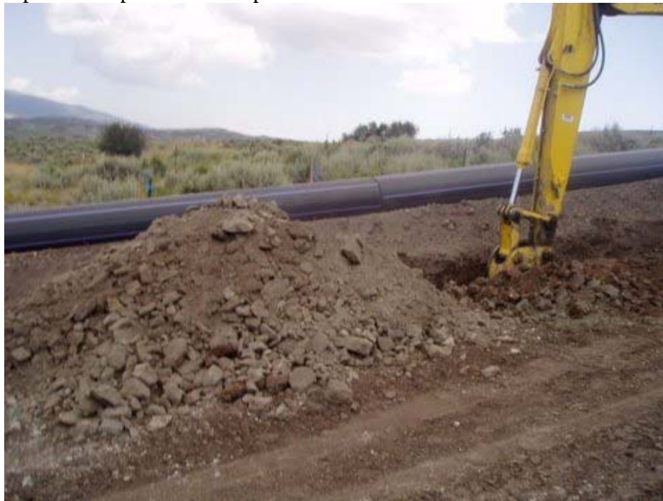
Pipeline test pit excavation pictures.
