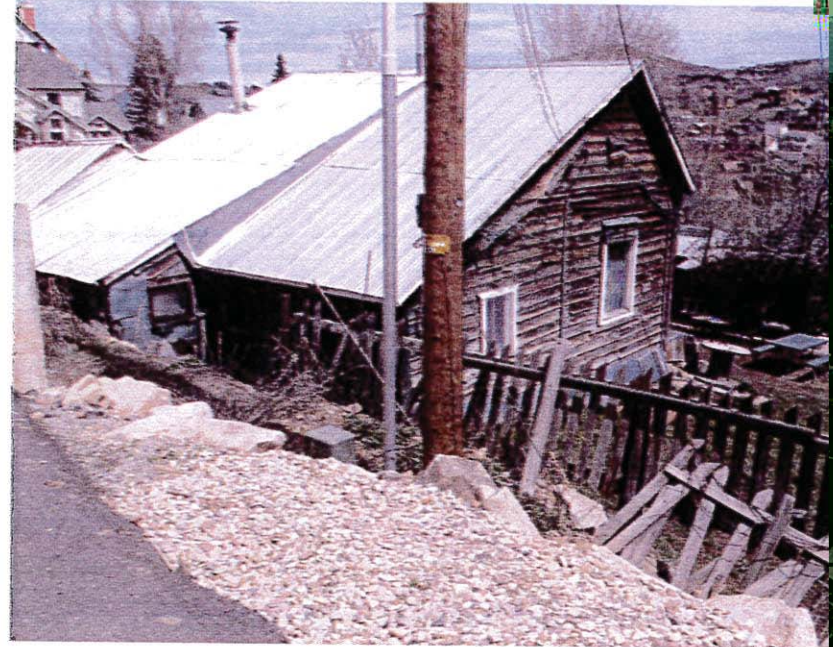
VIEW OF HOME FROM DRIVEWAY
