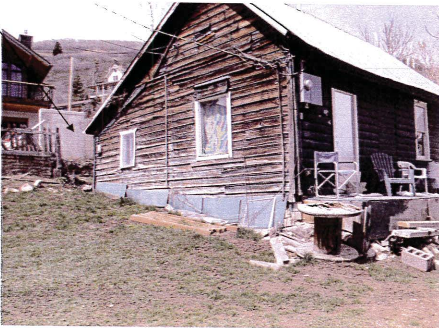
BACK AND SIDE VIEW & RETAINING WALL
