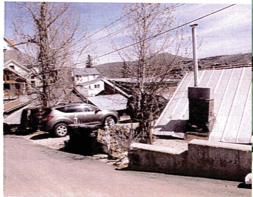
DRIVEWAY RETAINING WALL
