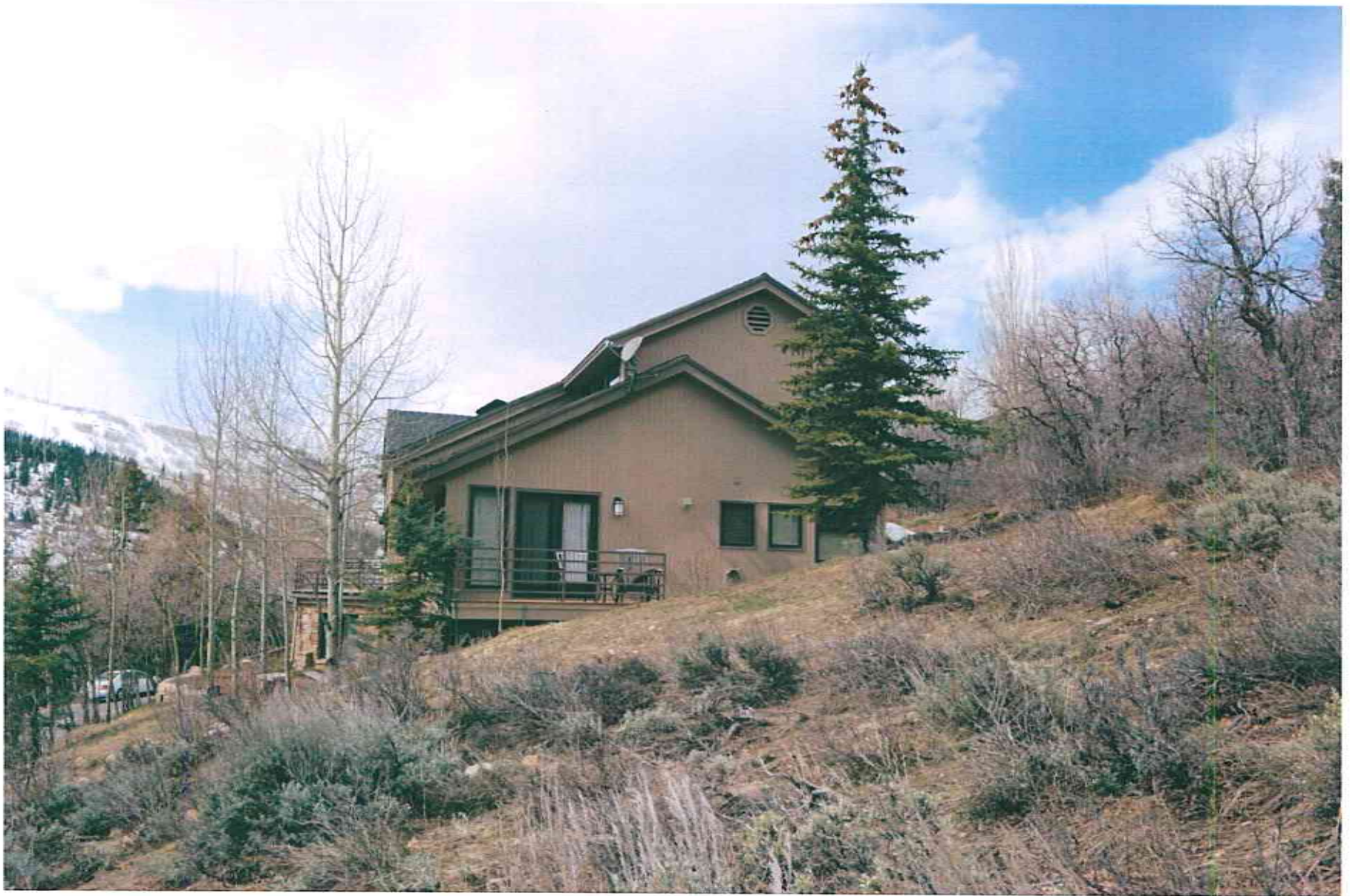
Sunnyside, Lot 11 – looking west
