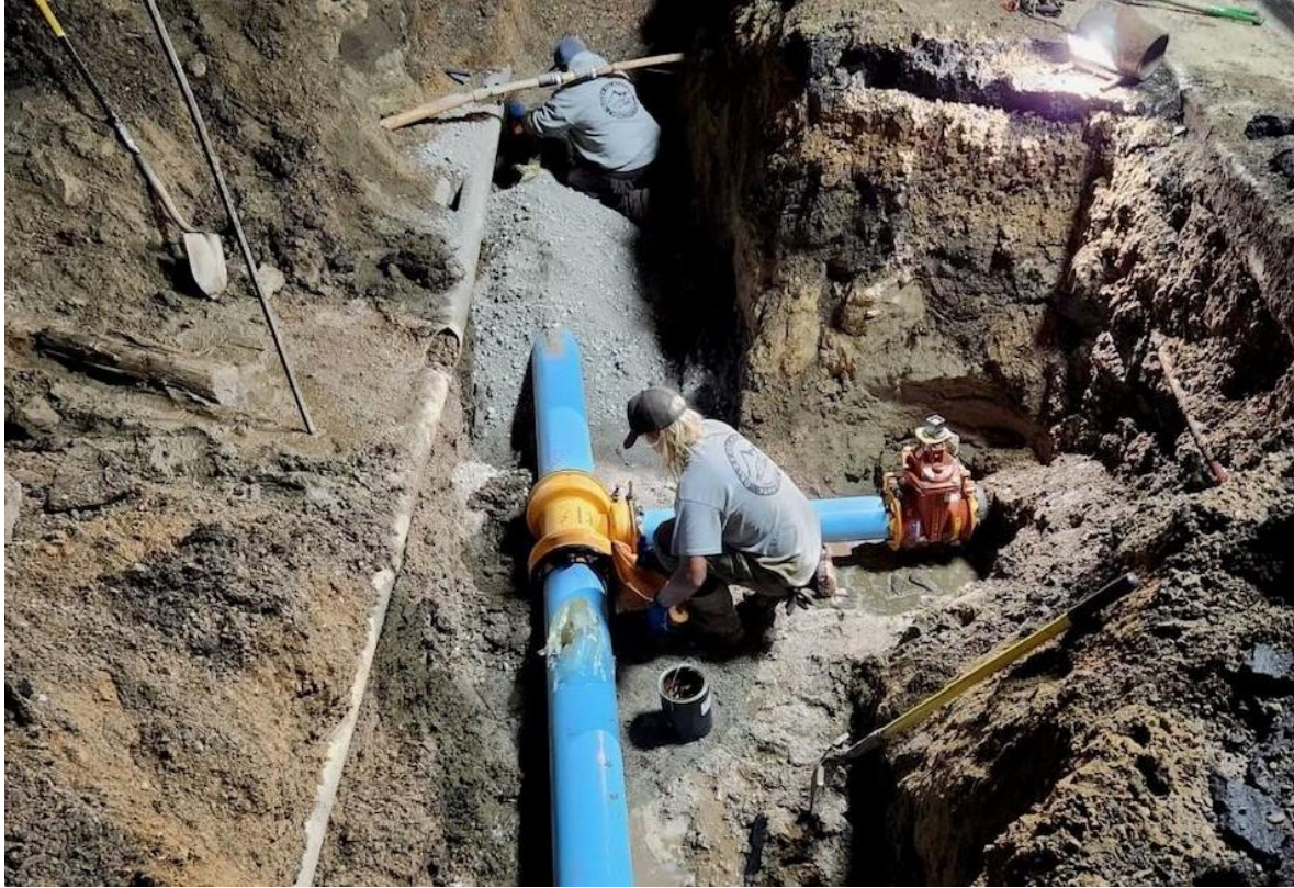
Figure 6, Main Street Water Line Repair. Source: PCMC, as of August 2023.
