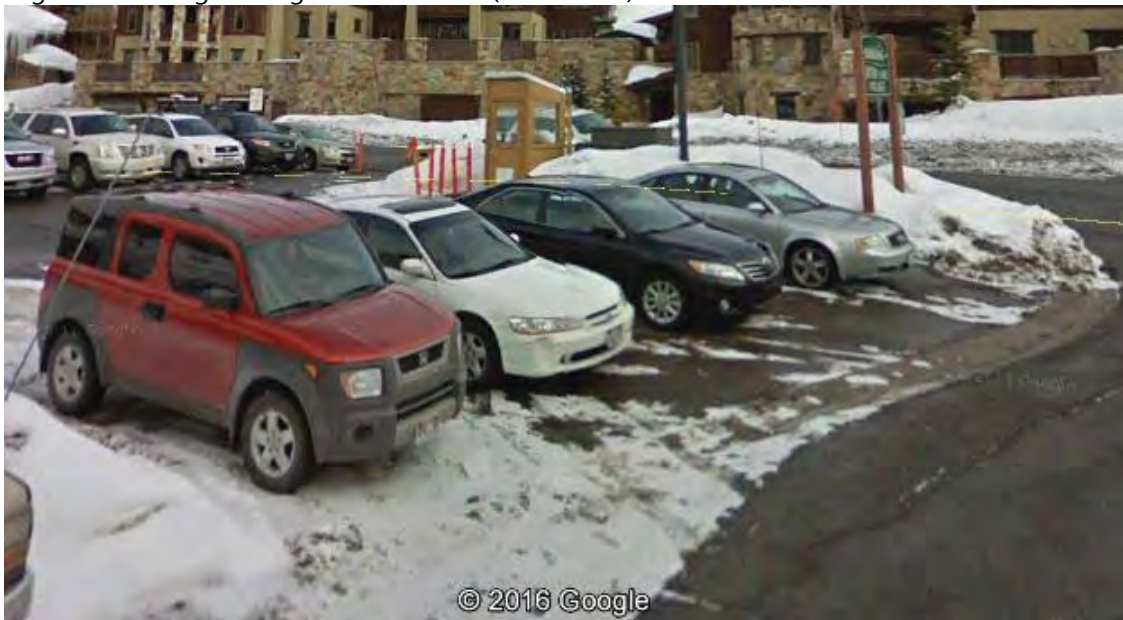
Figure 2: Existing Parking Lot Conditions (rolled curb)
