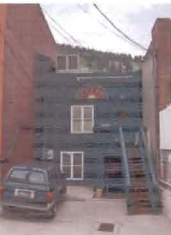
Rear View Park City Jewelers Building
