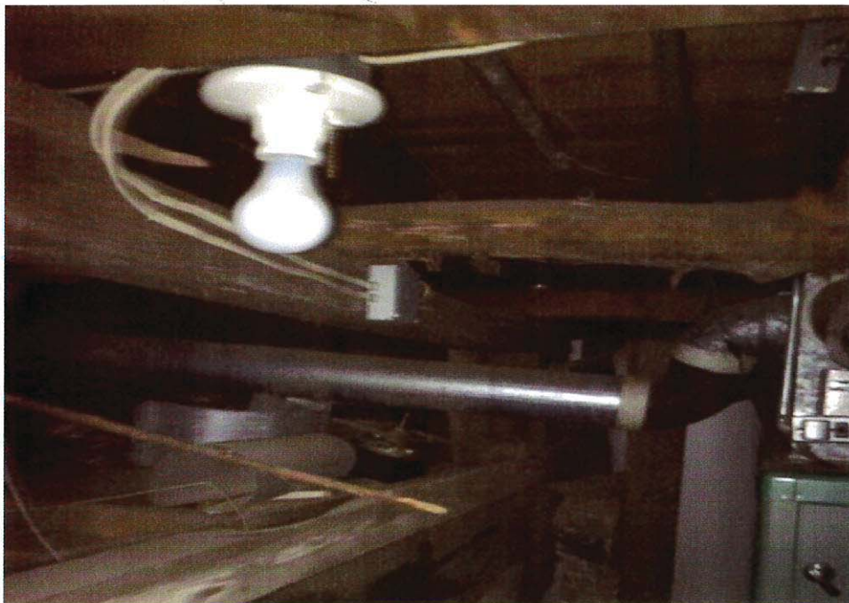
Photo 6: Sub-Floor Beams and Joists
