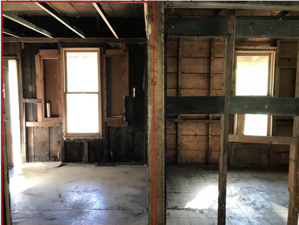
Figure 3: Photo looking to the front (east) of the house where the original exterior wall (middle of photo) partitions the addition (right of photo) dated circ. 1930s-40s.
