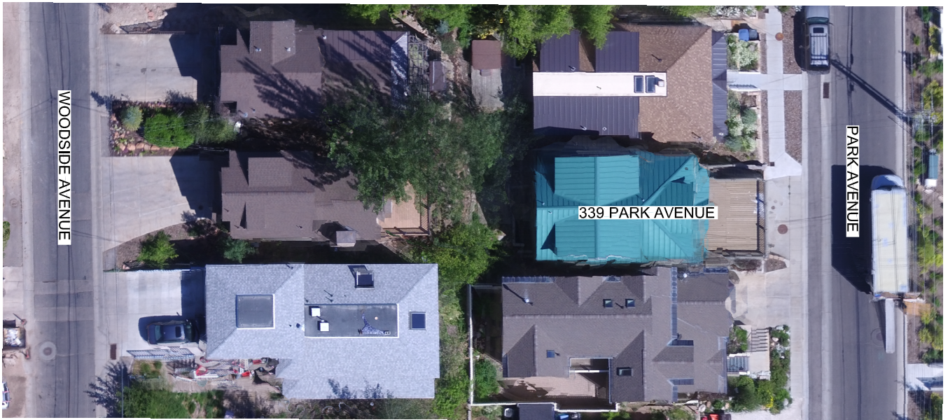
EXISTING / SURROUNDING STRUCTURES AND PROPERTIES
