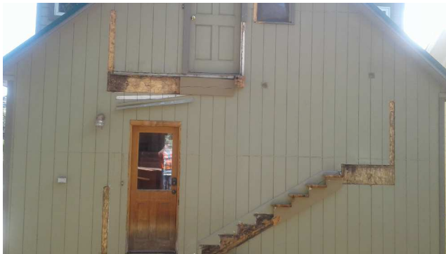
SECOND AND THIRD FLOOR REAR ENTRANCES
