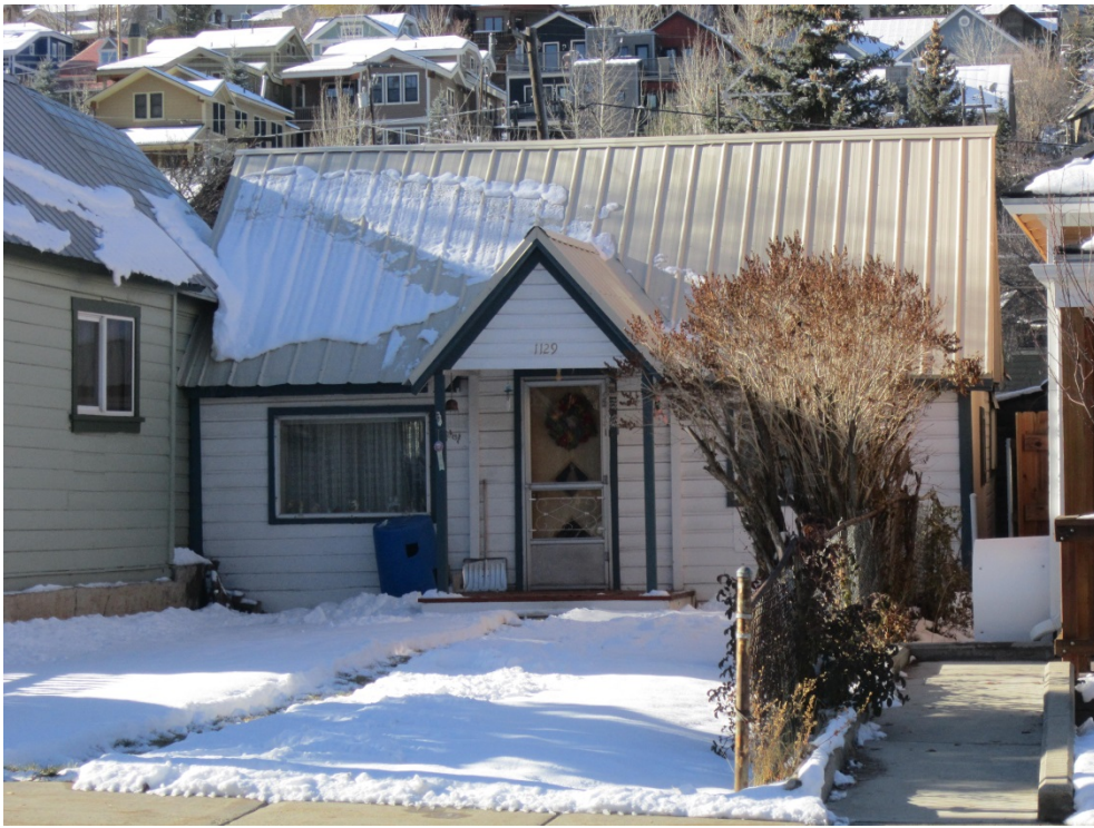
1129 Park Avenue. Northeast oblique. November 2013.
