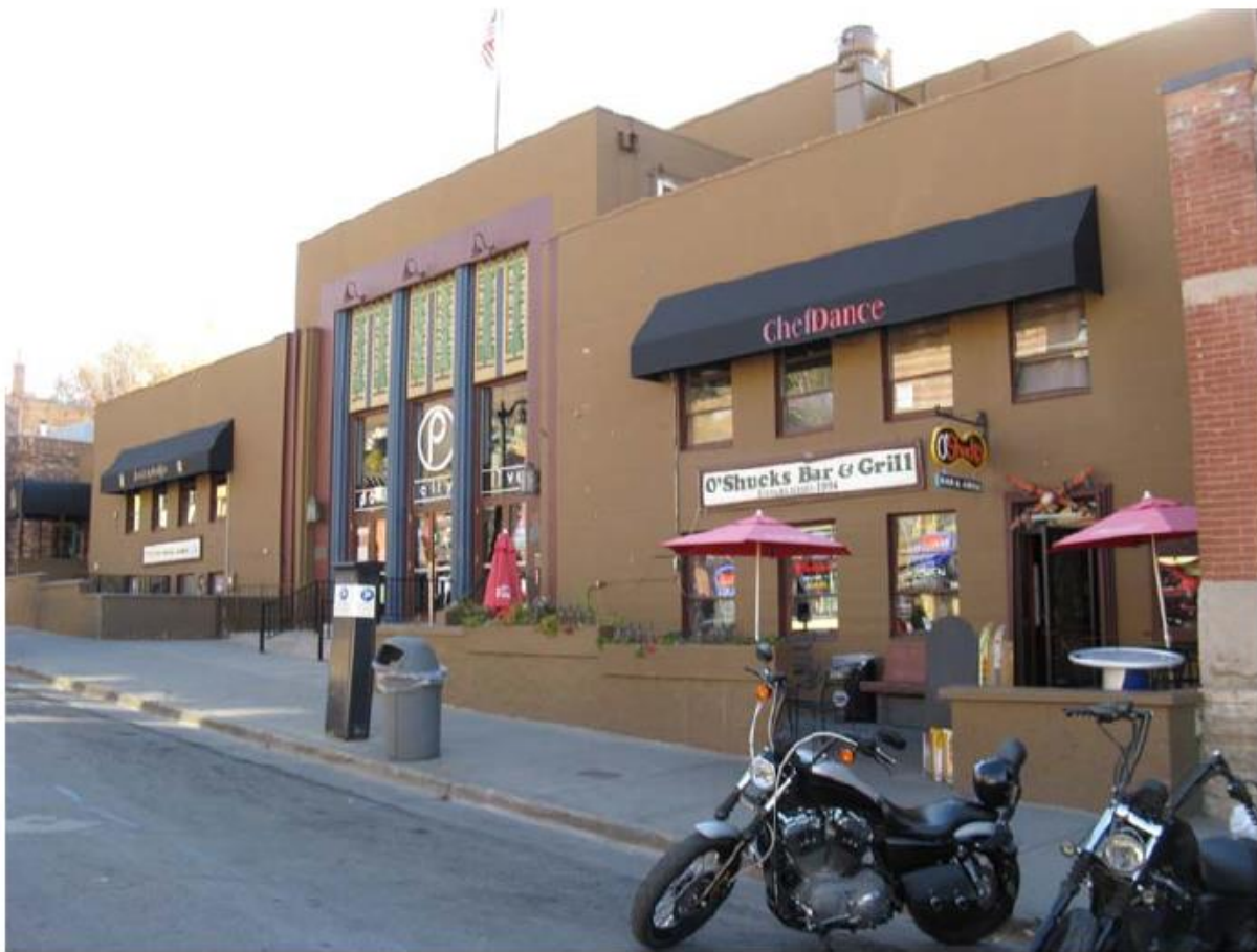
427 Main Street. Northeast oblique. October 2013.
