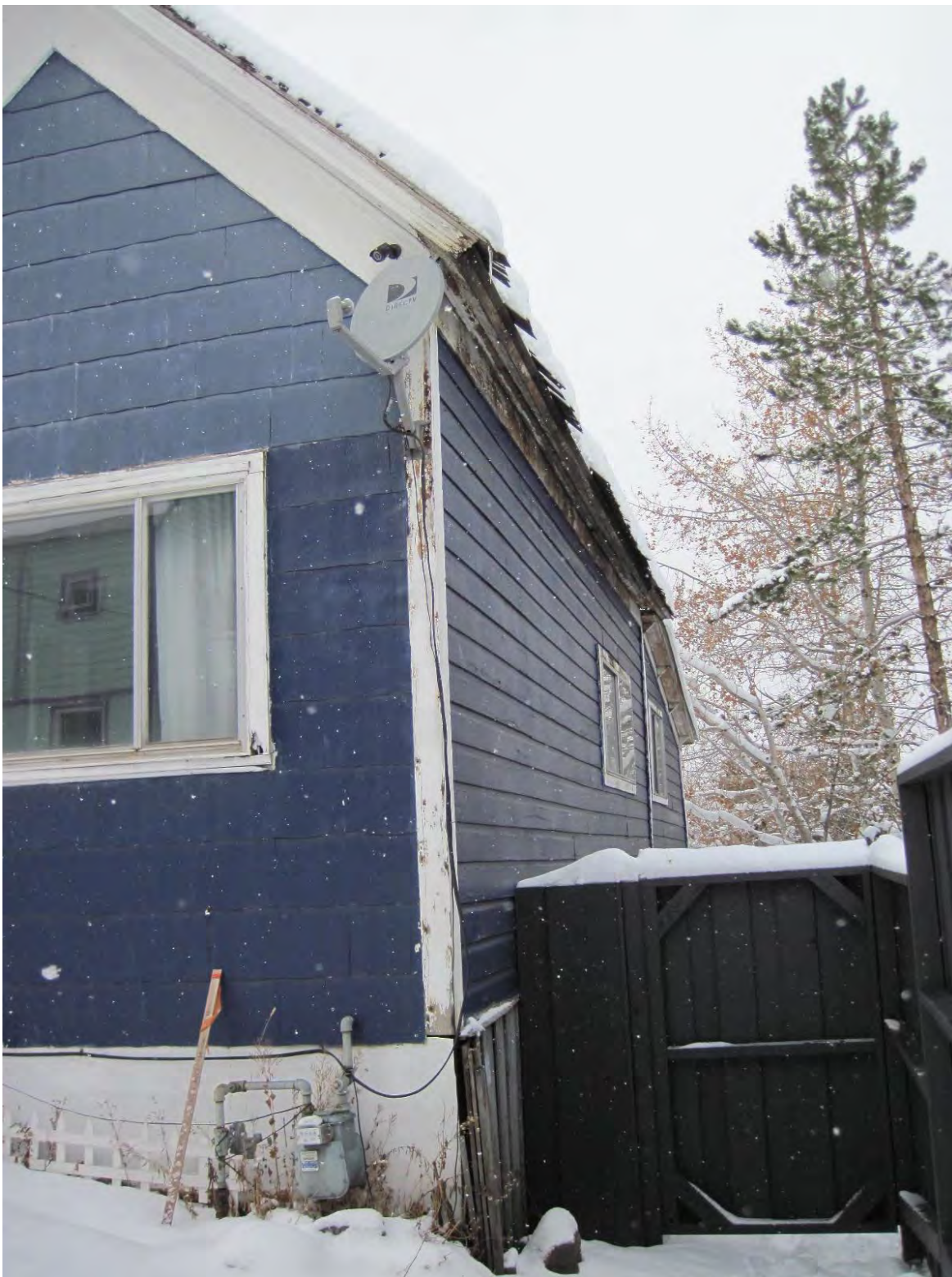
Photo 13: South / East elevation
