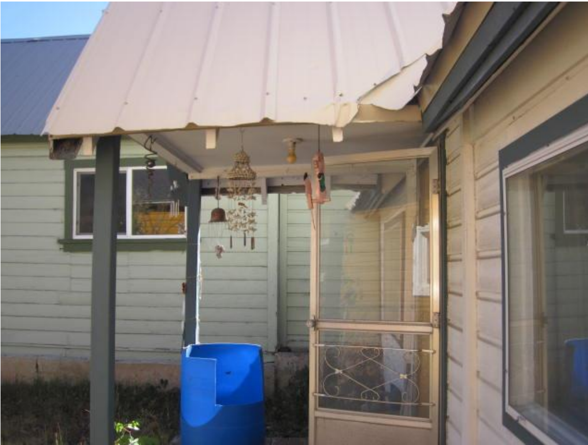
Photo 8: Covered entry porch, East elevation
