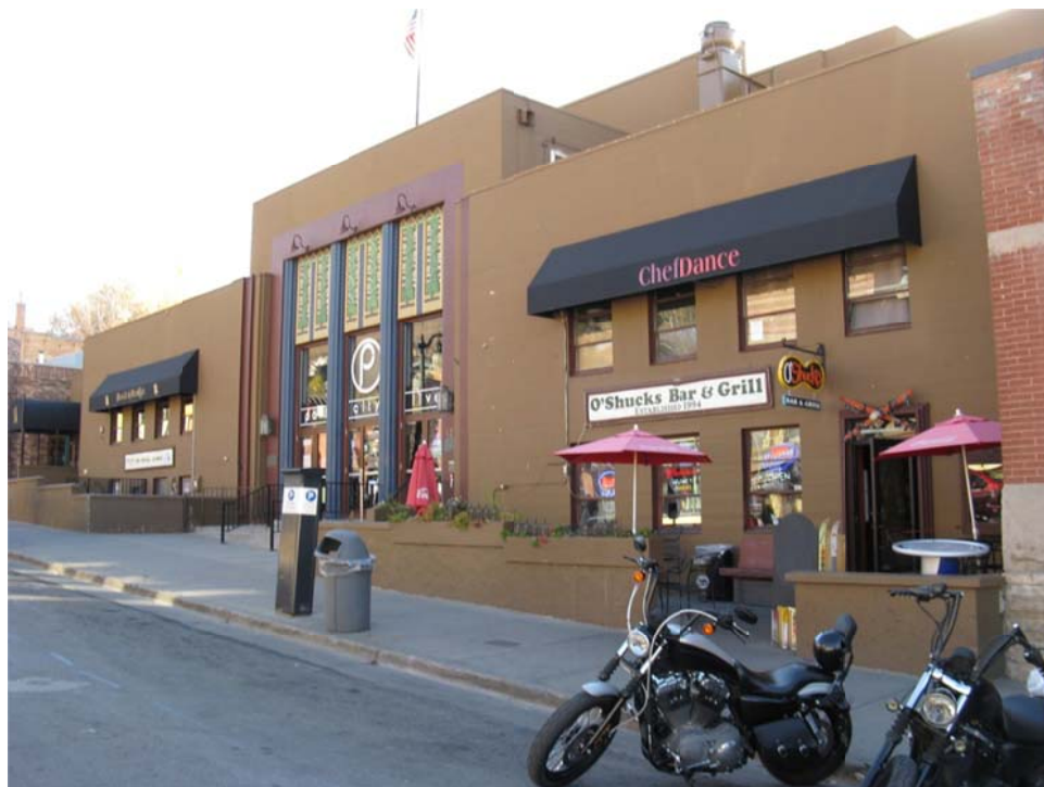
427 Main Street. Northeast oblique. October 2013.
