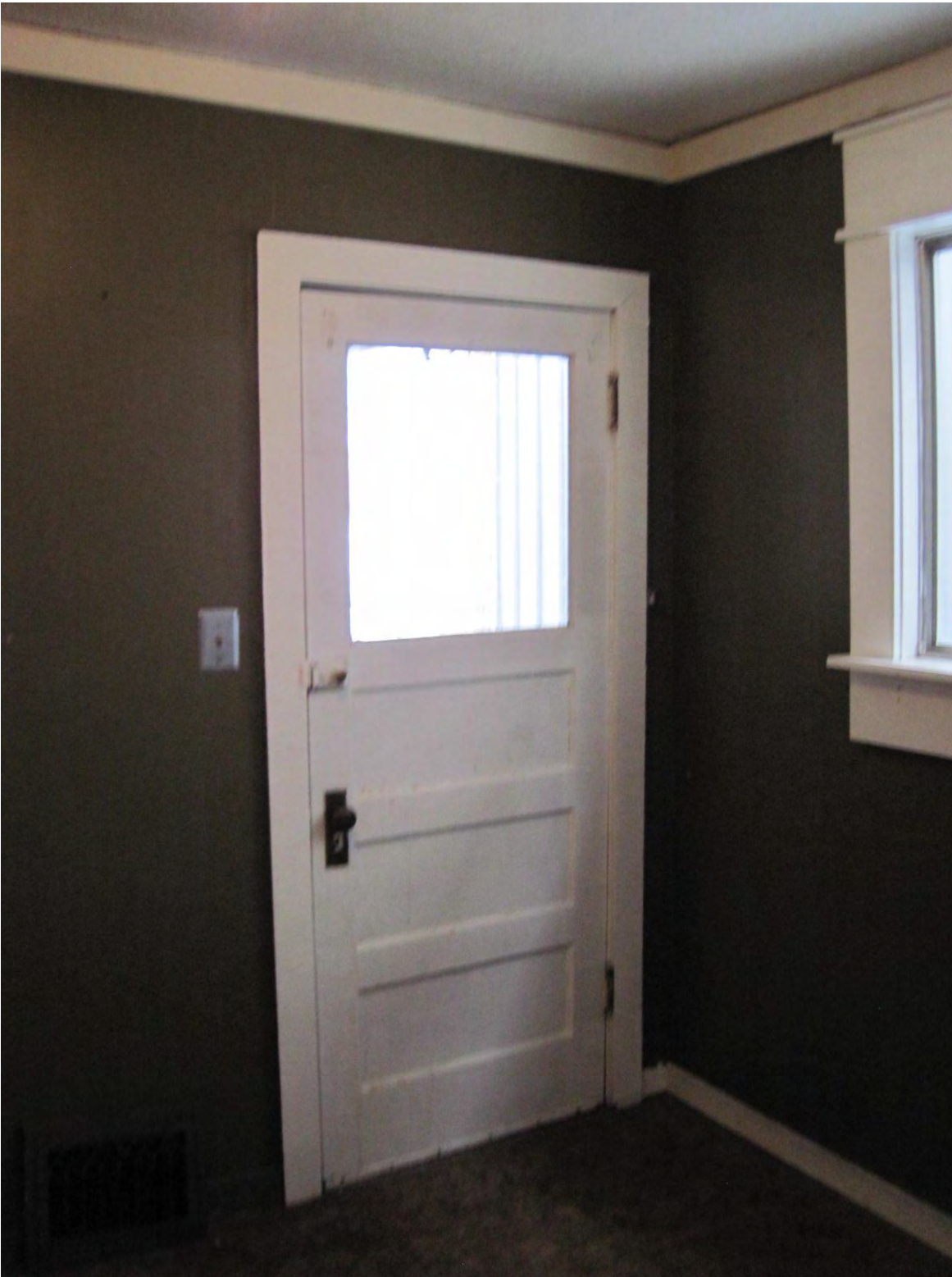
Photo 31: Entrance door at kitchen
