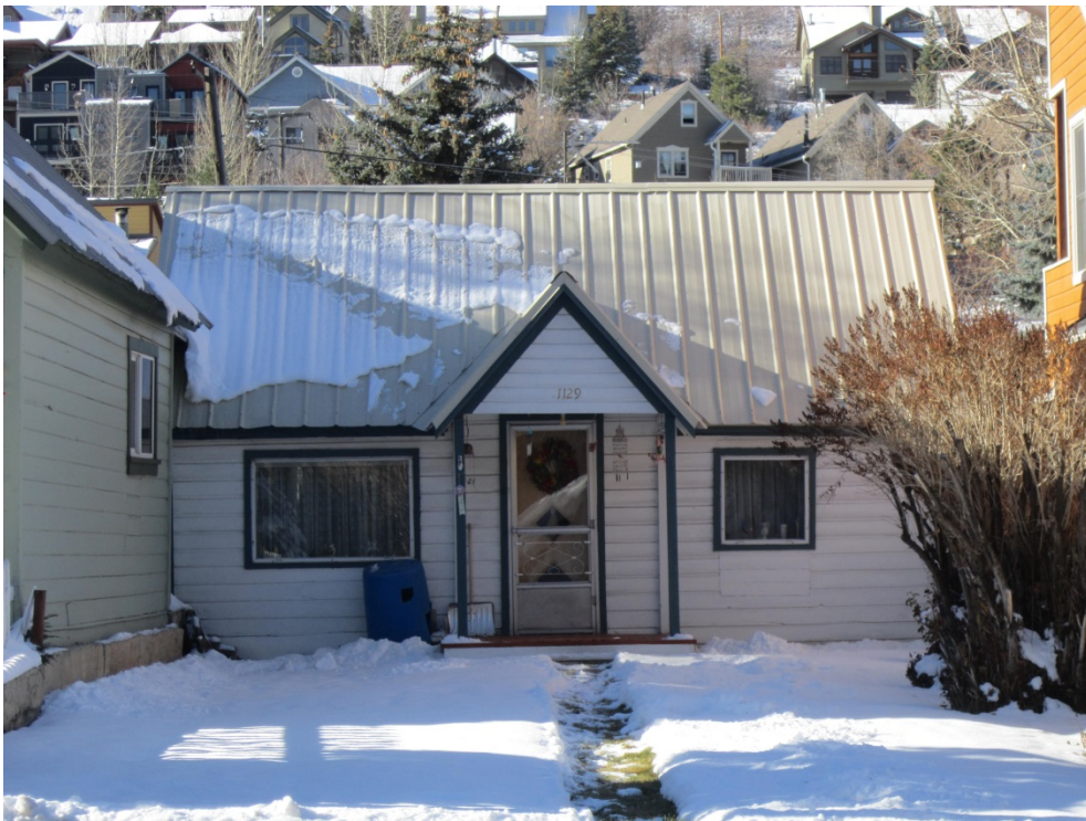
1129 Park Avenue. East elevation. November 2013.
