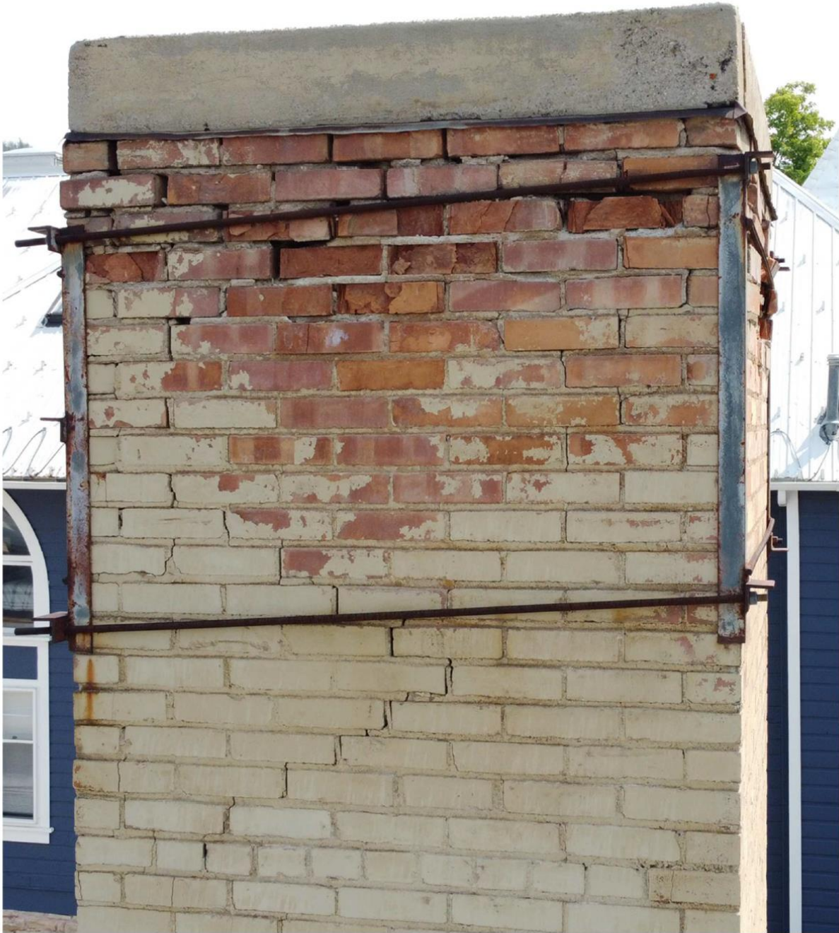
Figure 3: Wall Cracking
