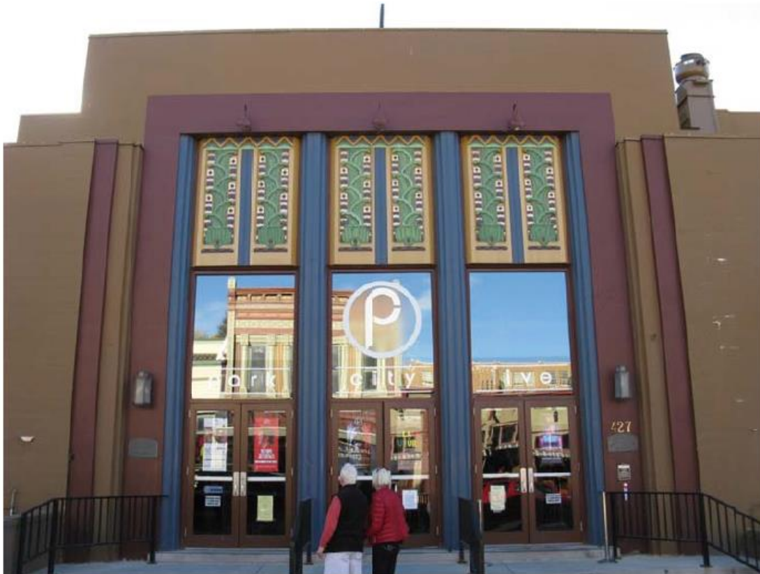
427 Main Street (main entrance). East elevation. October 2013.
