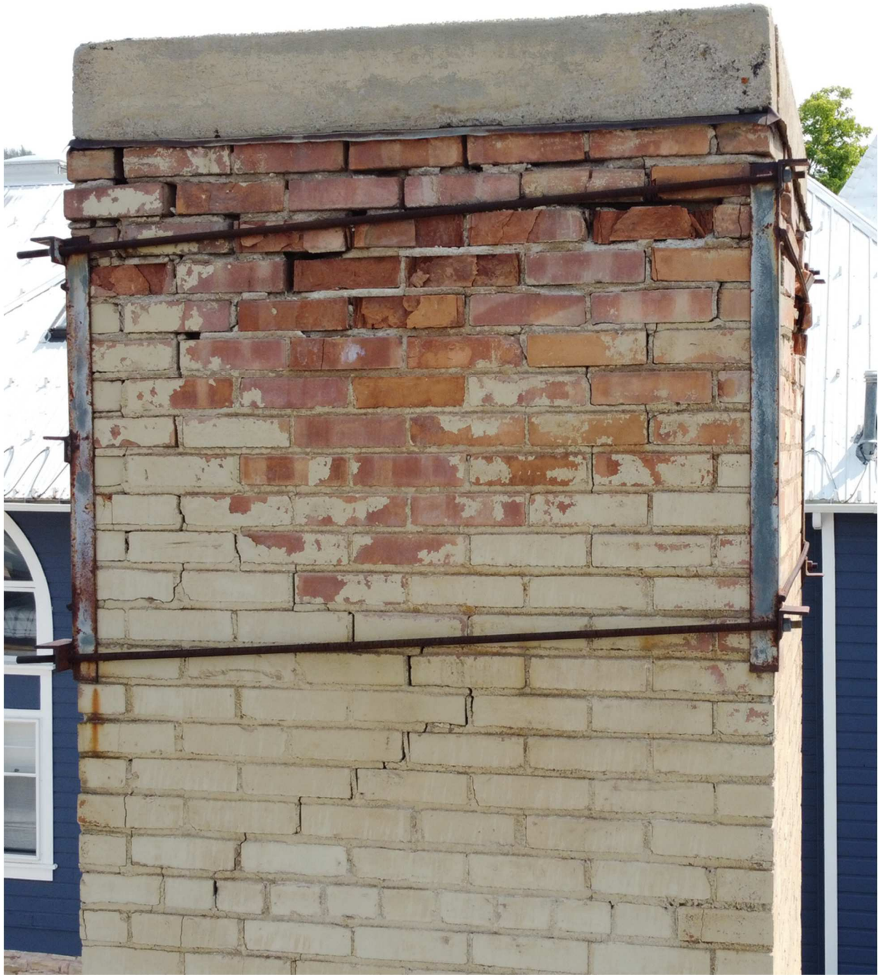
Figure 3: Wall Cracking
