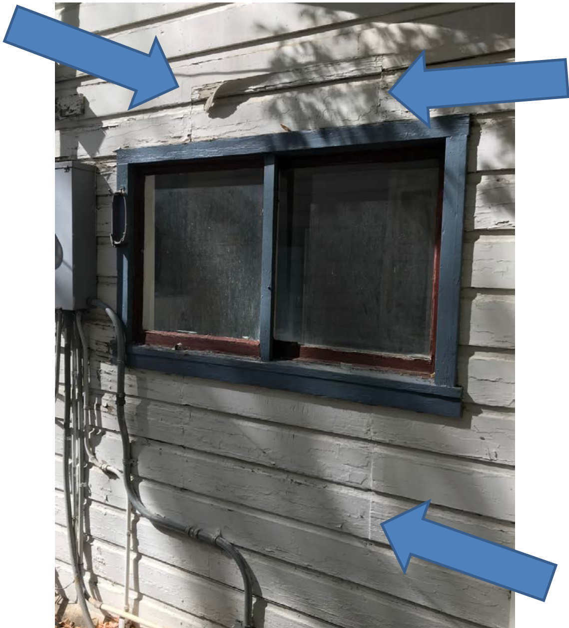
Image 6: South Elevation showing framed-in “ghost” window
