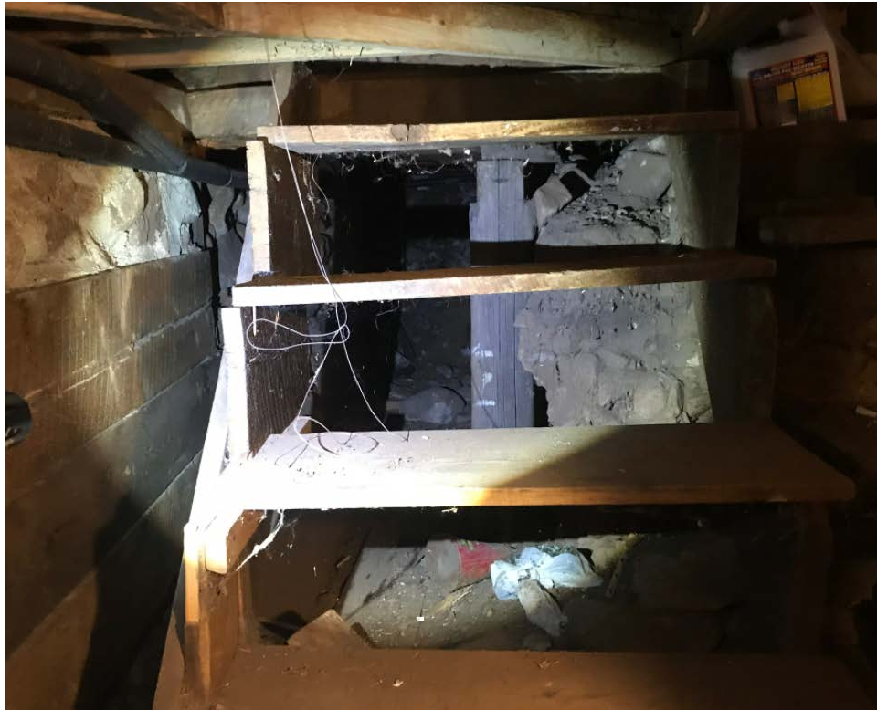
Image 8: Crawlspace looking south towards partially excavated area below historic shed addition (photo taken by staff).
