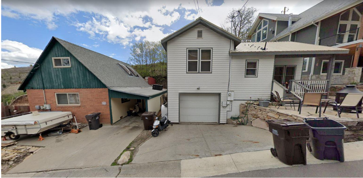
Figure 1. Image of 91 King Road (left) and 95 King Road (right), from Google Maps.
