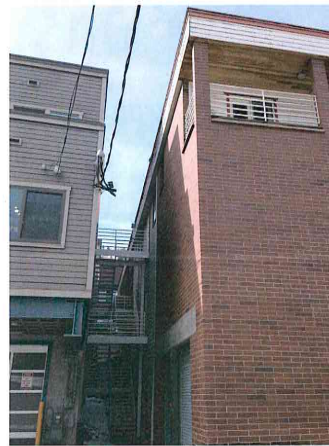
North Elevation Looking Toward Site
