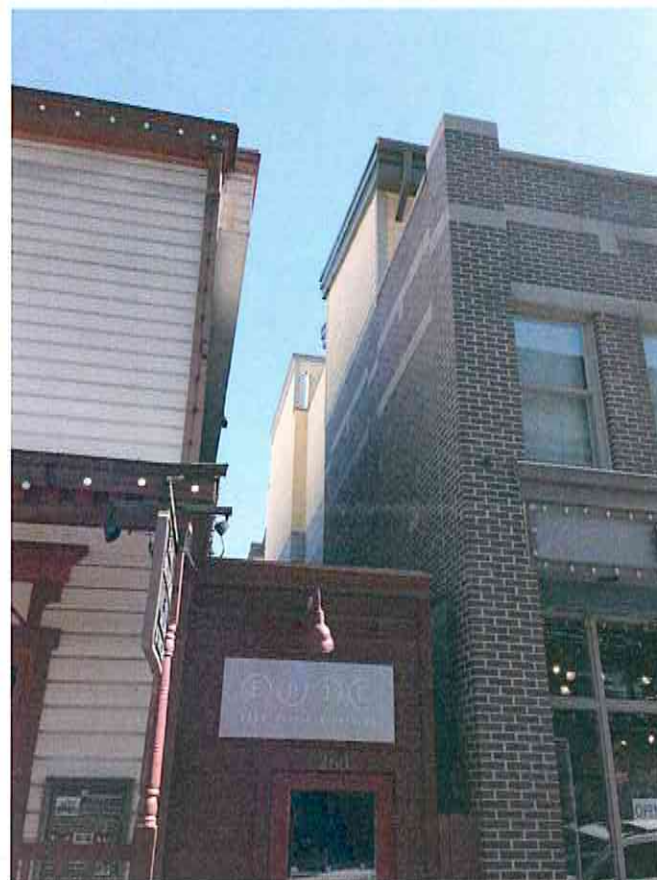
North Elevation Looking Toward Site
