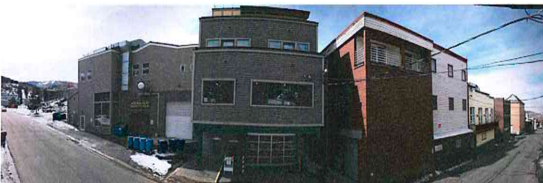
East Elevation Panorama Looking Toward Site
