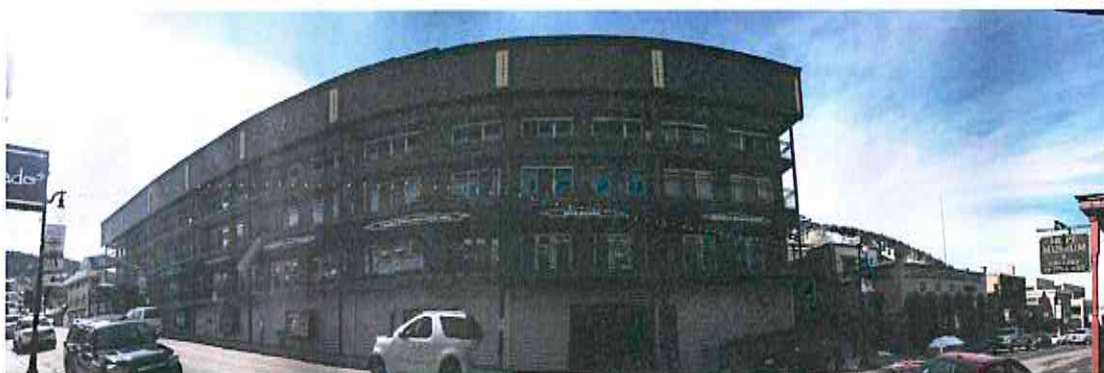
West Elevation Panorama Looking From Site
