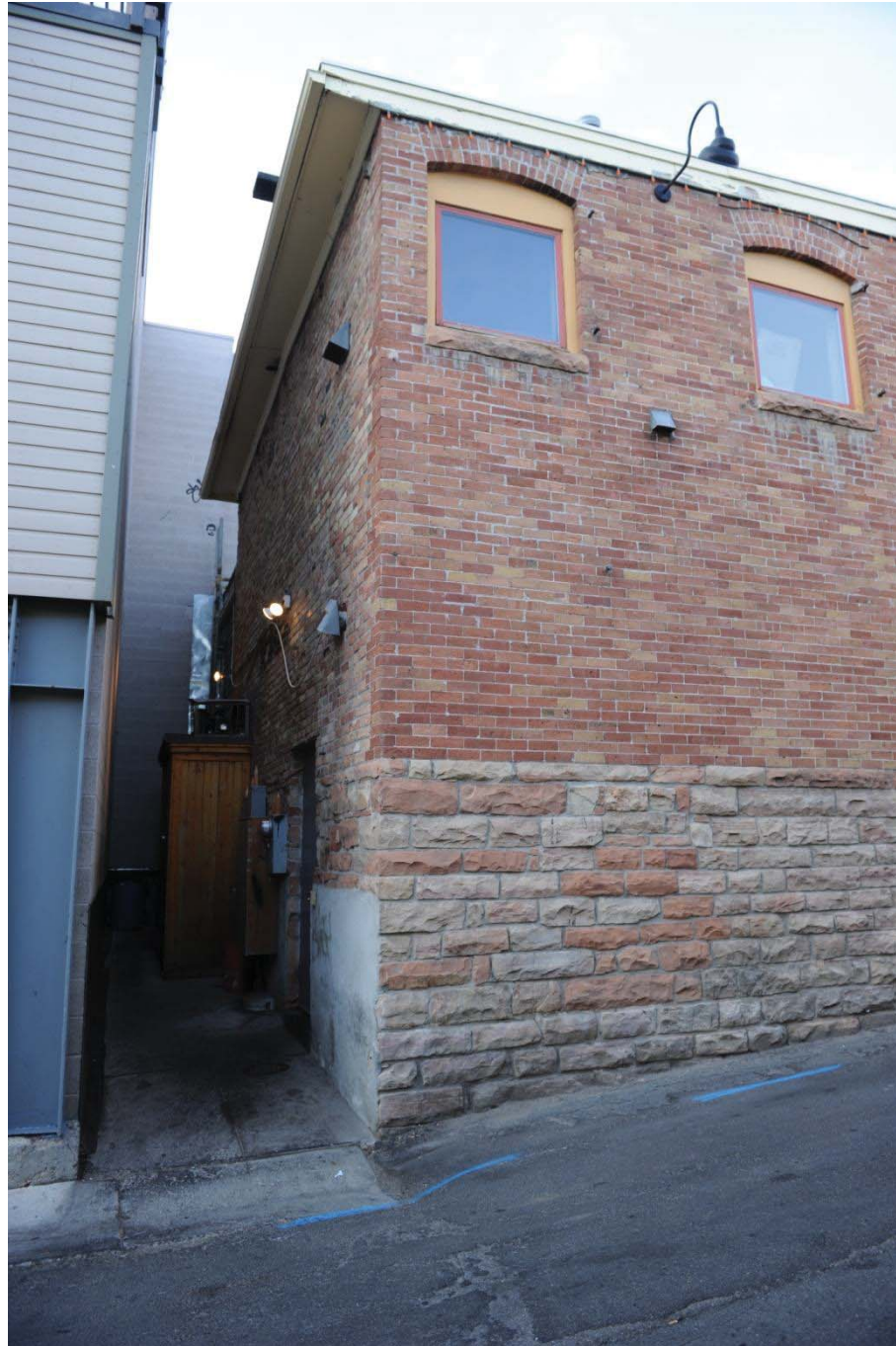
368 Main Street – looking southeasterly
