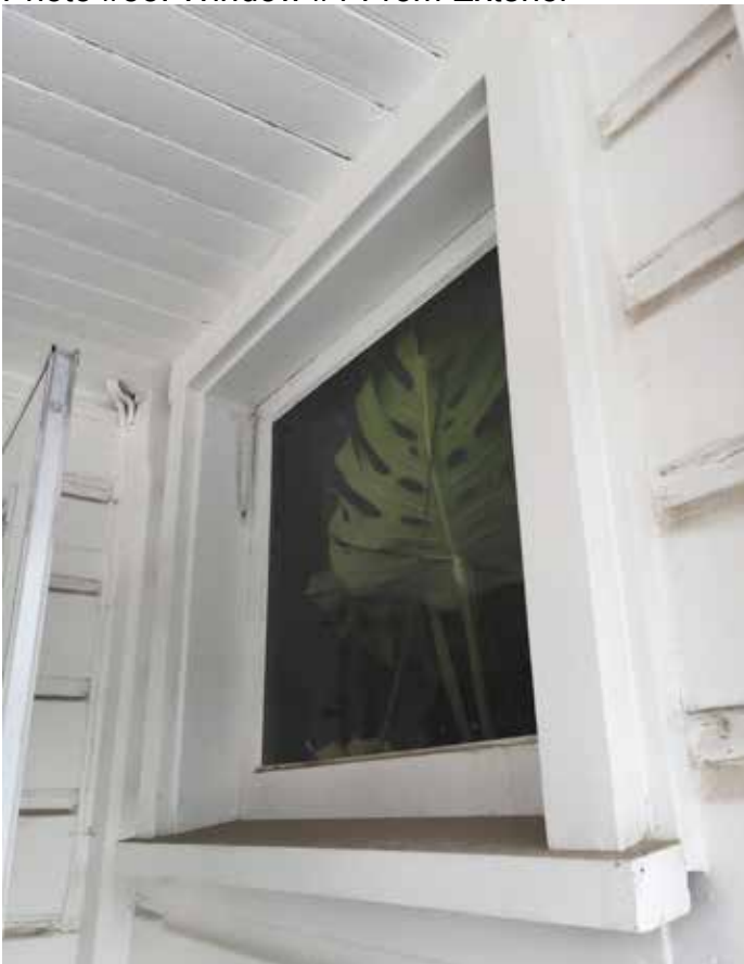
Photo #53: Window #1 From Exterior
