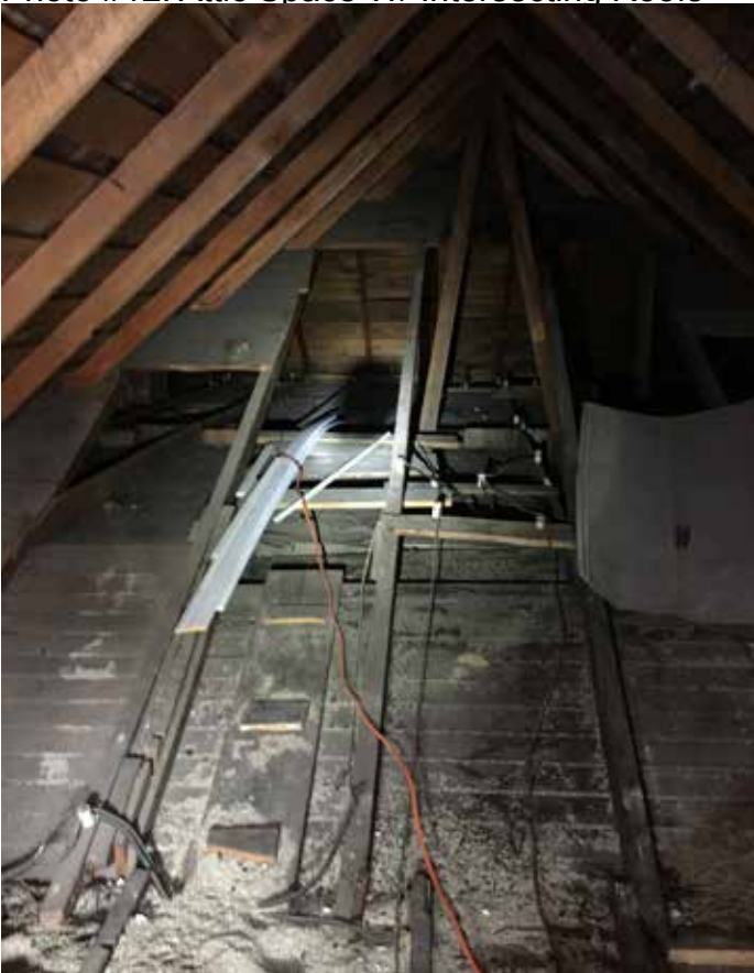
Photo #12: Attic Space W/ Intersecting Roofs
