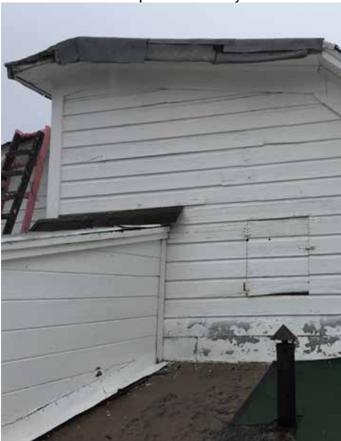
Photo #31: Close Up At Attic Entry
