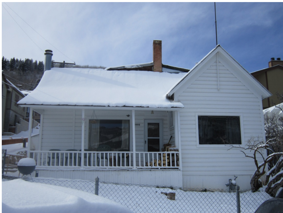
1003 Norfolk Avenue. East elevation. November 2013.
