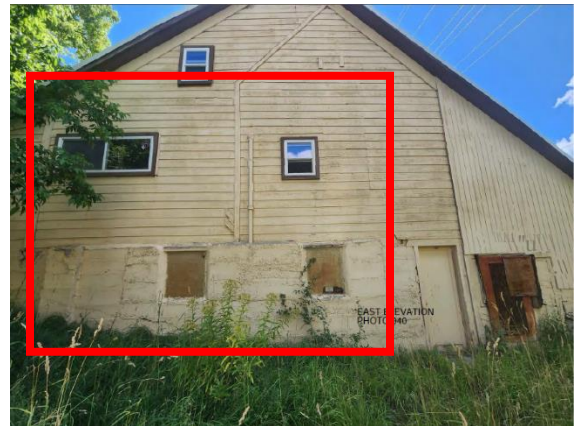
Figure 5: Photograph of eastern facade of home showing area of siding proposed to be removed.
