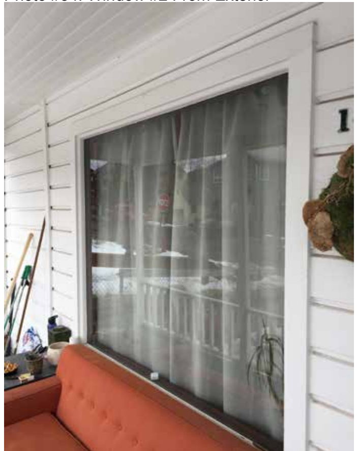
Photo #54: Window #2 From Exterior
