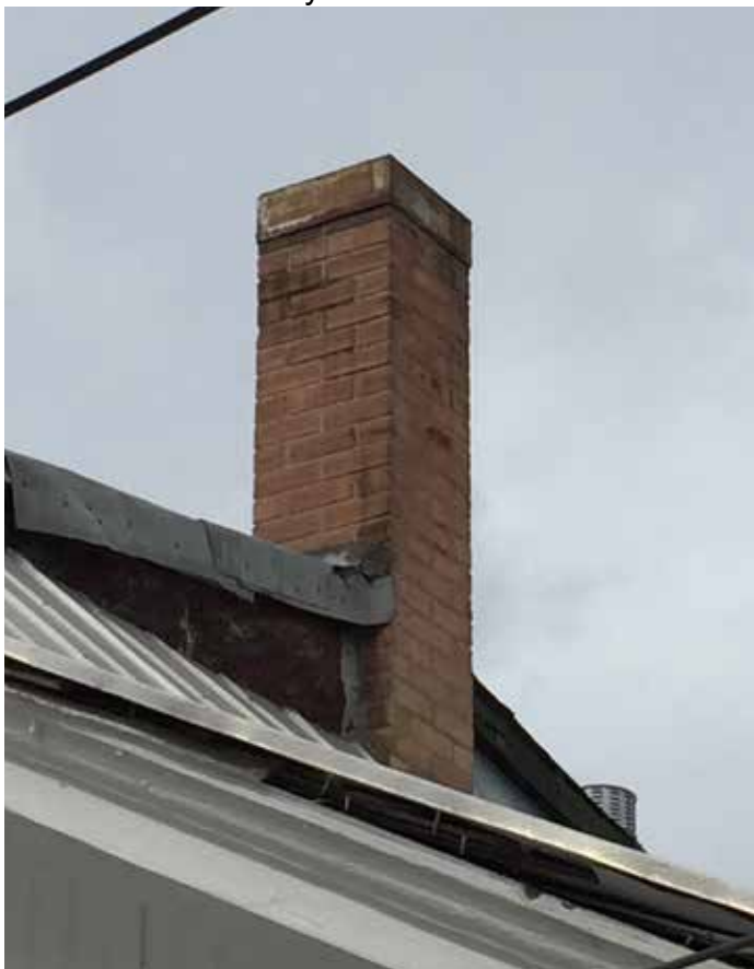
Photo #19: Chimney From Southeast
