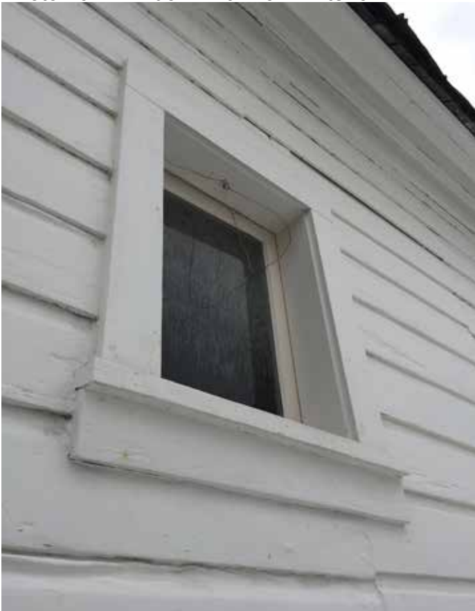
Photo #62: Window #10 From Exterior
