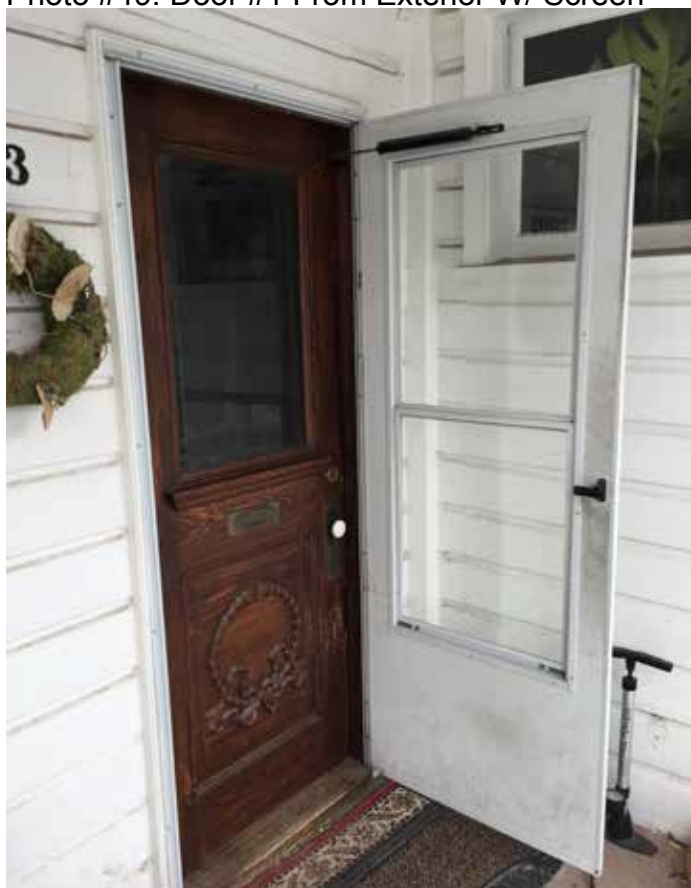
Photo #49: Door #1 From Exterior W/ Screen
