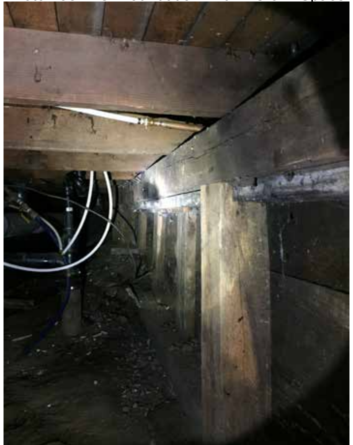
Photo #38: T.O. Foundation Within Crawl Space
