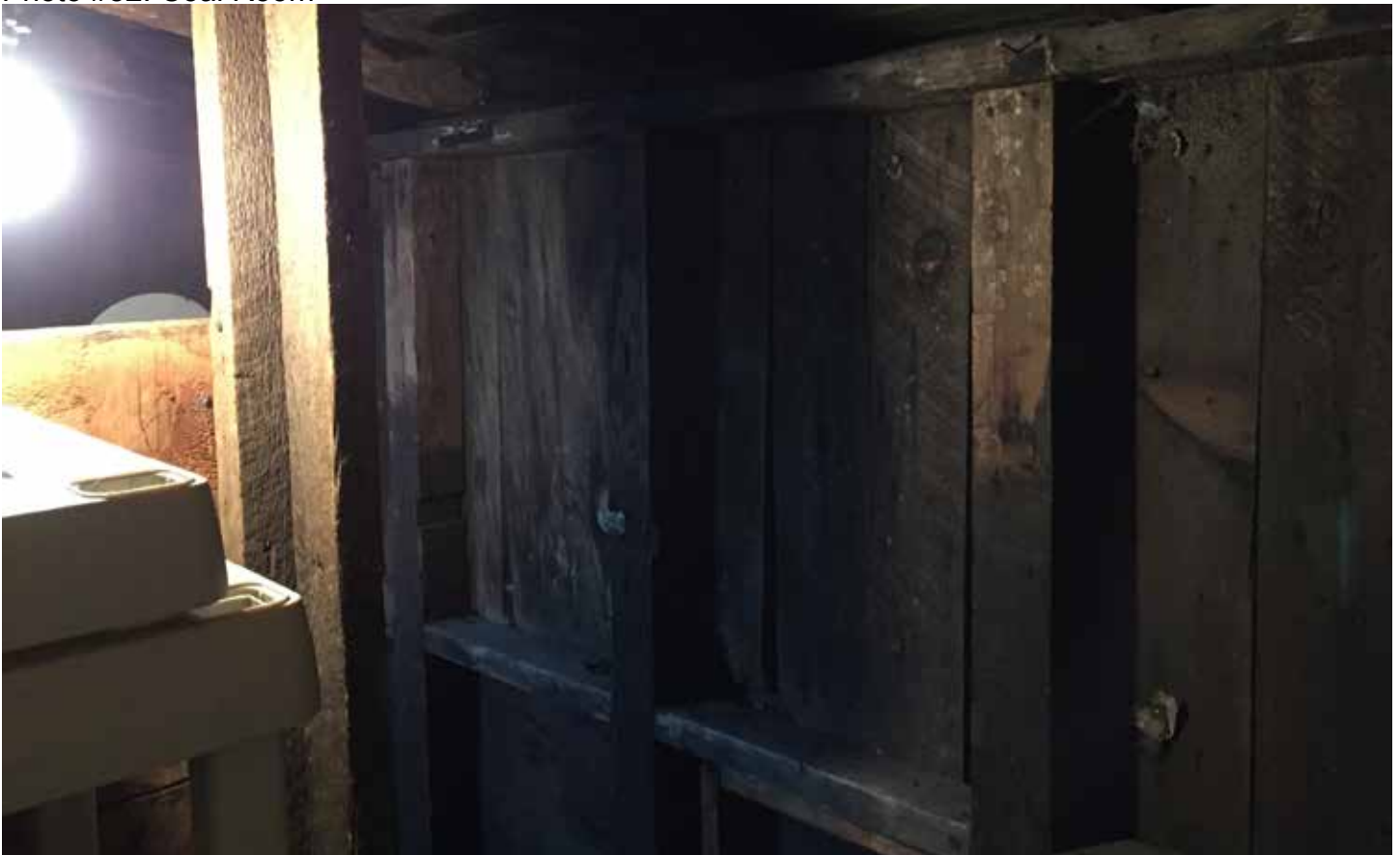
Photo #82: Coal Room
