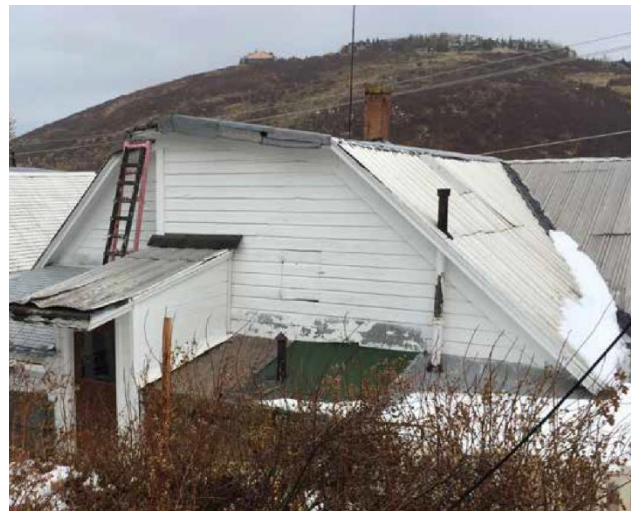
Figure 4: Photo of rear of roof; overbuilt gambrel form
