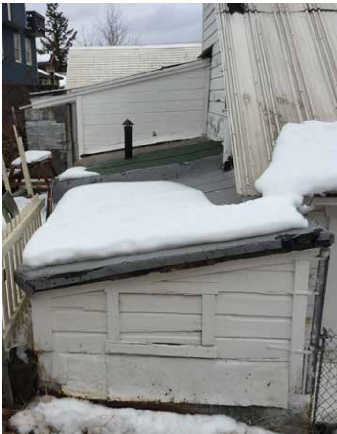
Photo #16: Roofs Over Coal/Storage/Rear Entry
