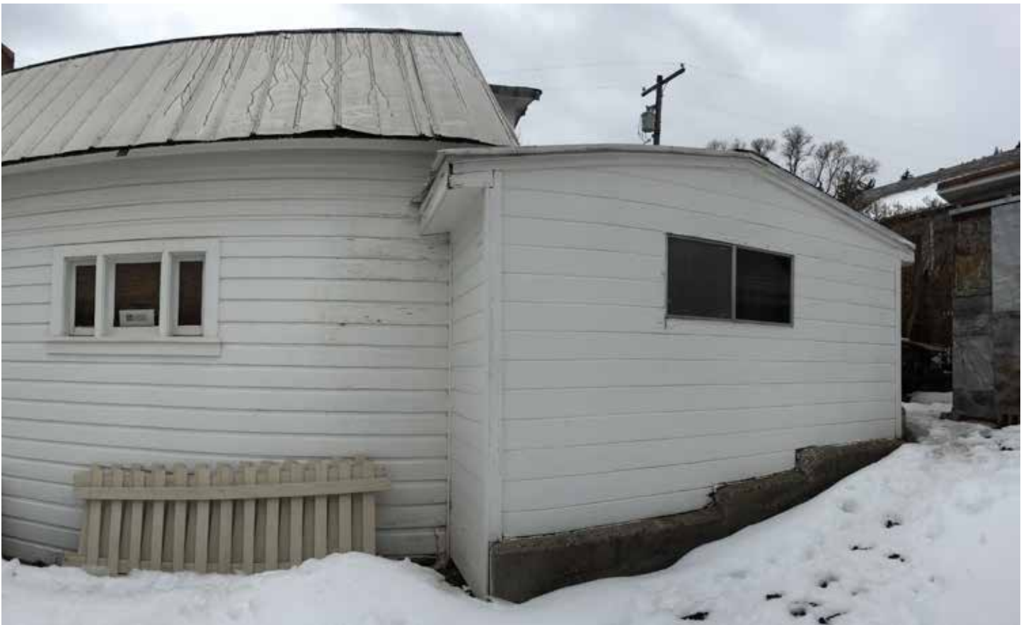
Photo #34: North Facade
