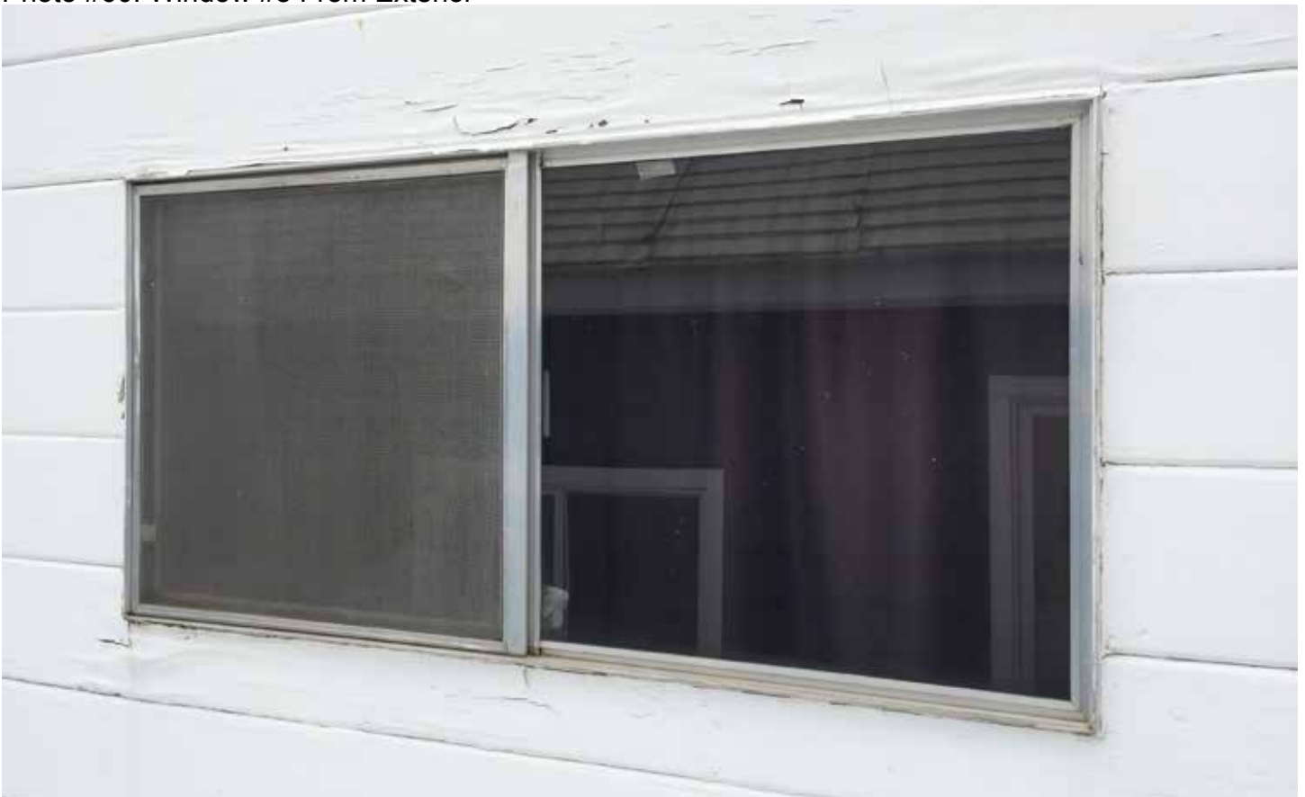
Photo #60: Window #8 From Exterior
