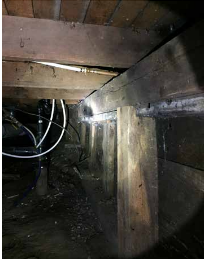
Photo #38: T.O. Foundation Within Crawl Space
