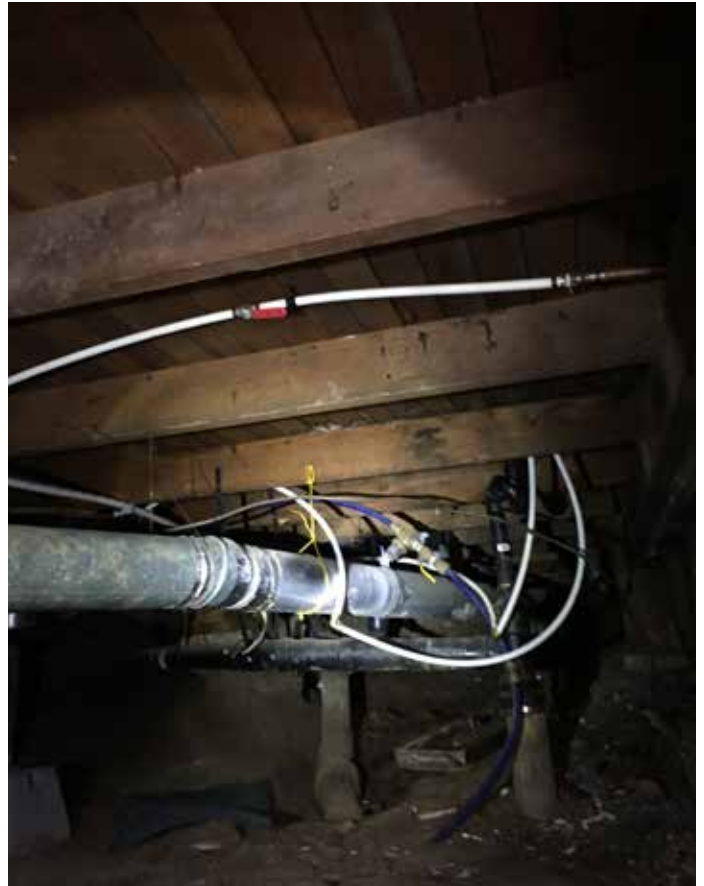
Photo #11: B.O. 2x8 Main Floor Structure
