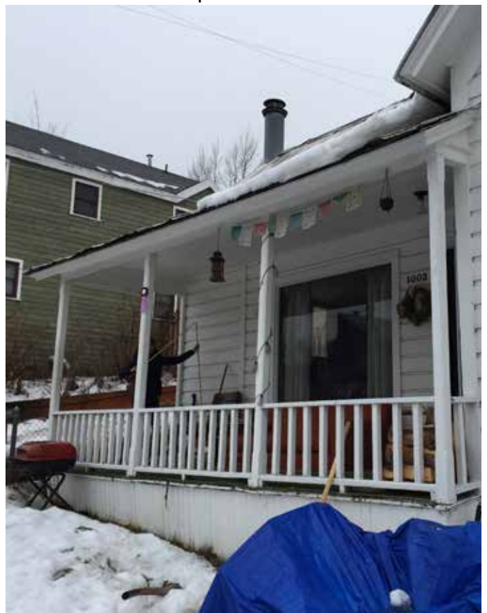
Photo #27: Close Up At Porch
