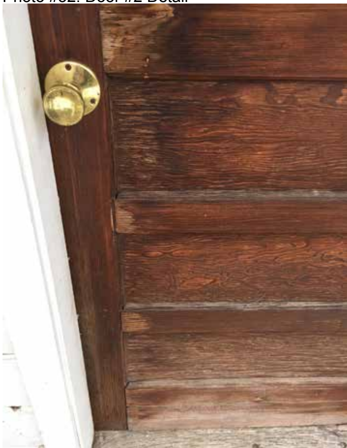
Photo #52: Door #2 Detail
