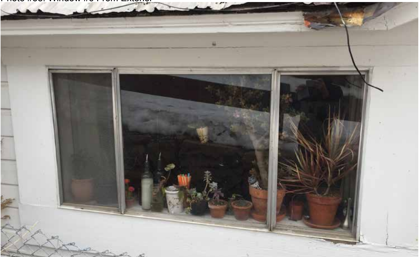
Photo #58: Window #6 From Exterior
