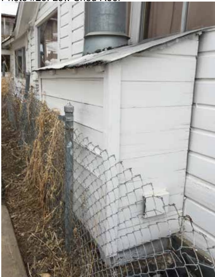
Photo #23: Low Shed Roof
