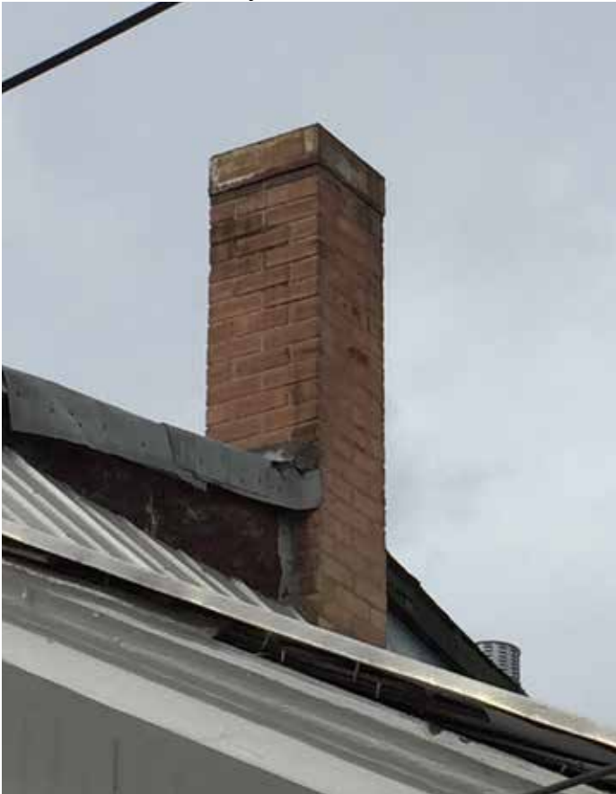
Photo #19: Chimney From Southeast
