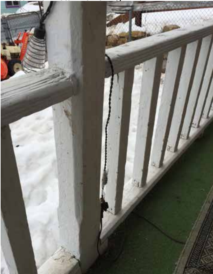
Photo #40: Detail At Railing
