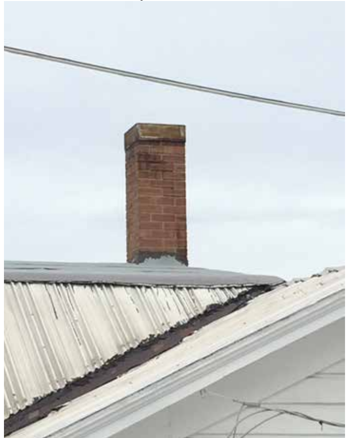
Photo #20: Chimney From South
