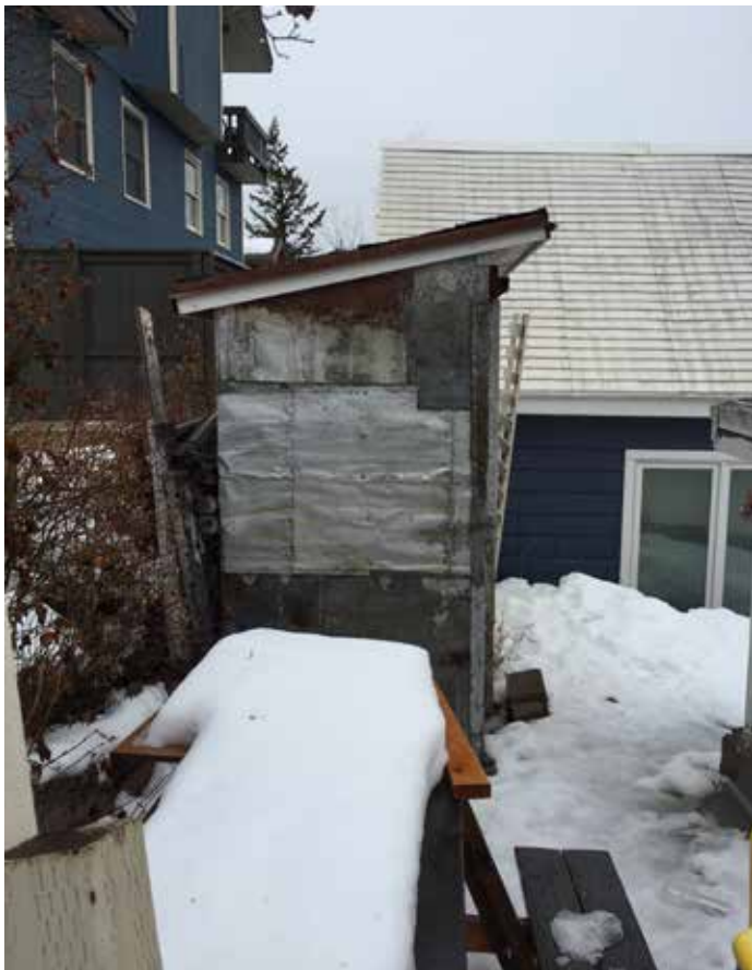
Photo #5: Shed Structure at Northwest Corner
