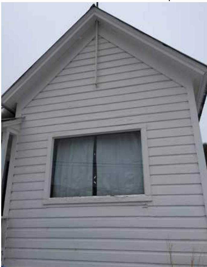
Photo #26: Gable Roofed Wall Close Up
