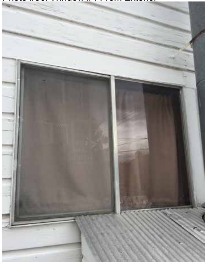
Photo #56: Window #4 From Exterior
