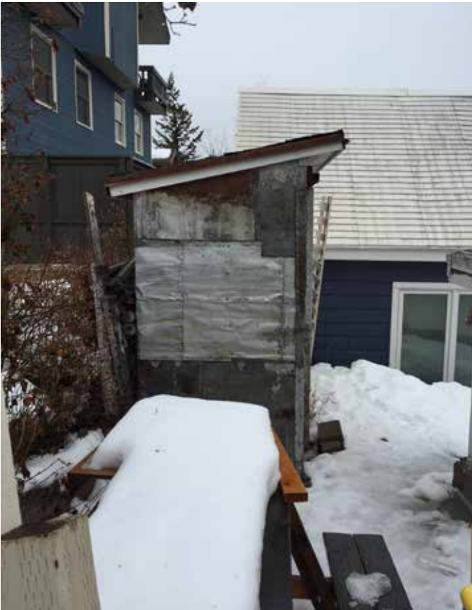
Photo #5: Shed Structure at Northwest Corner
