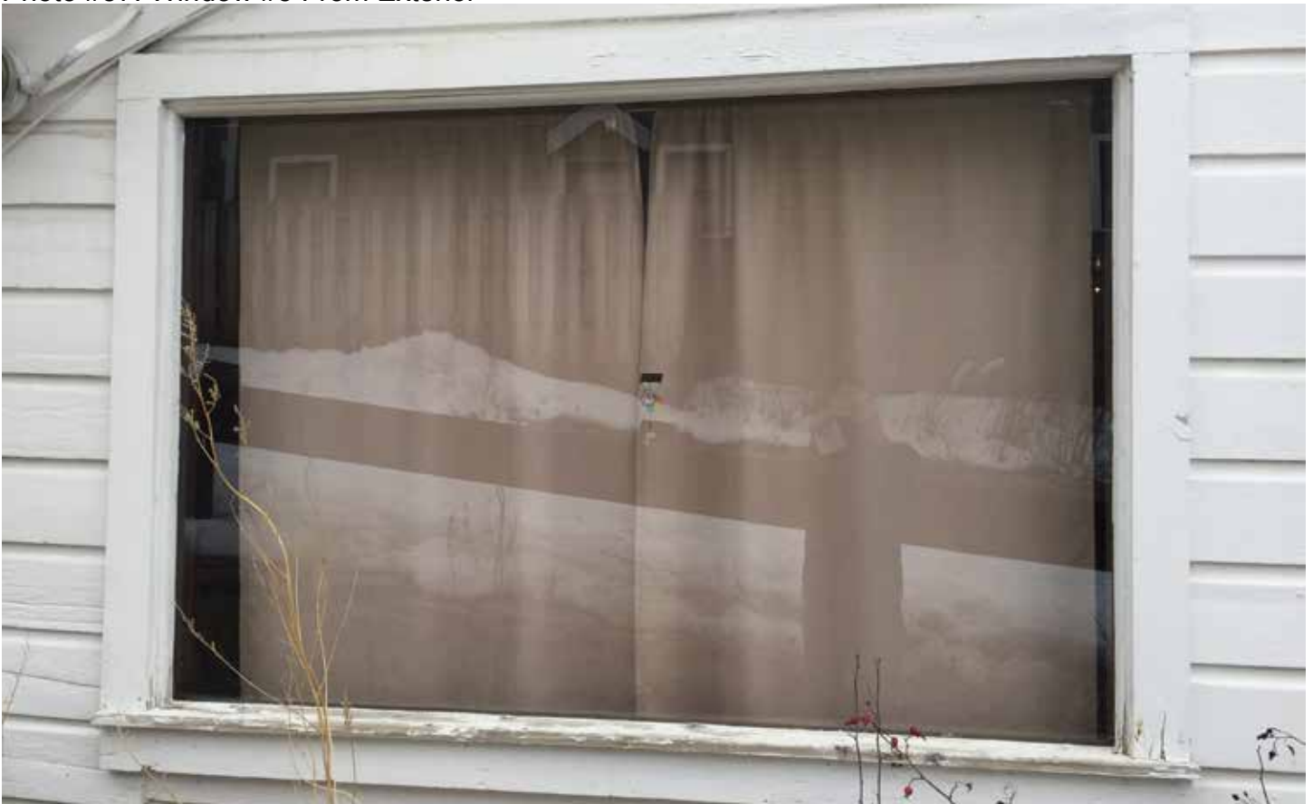
Photo #57: Window #5 From Exterior
