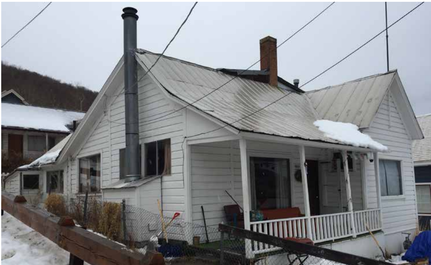
Photo #14: Original Roof Shape From Southeast Corner
