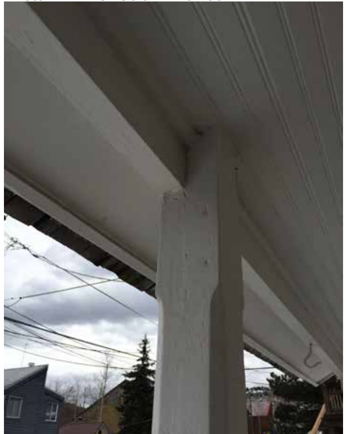
Photo #41: T.O. Column At Roof
