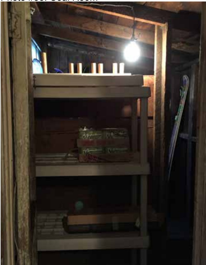
Photo #83: Coal Room
