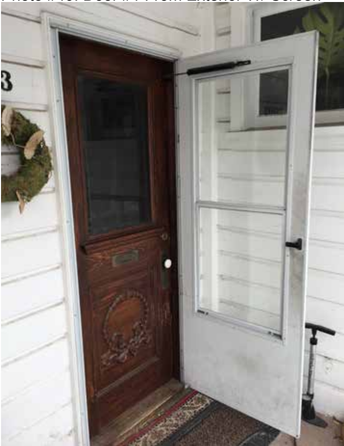
Photo #49: Door #1 From Exterior W/ Screen
