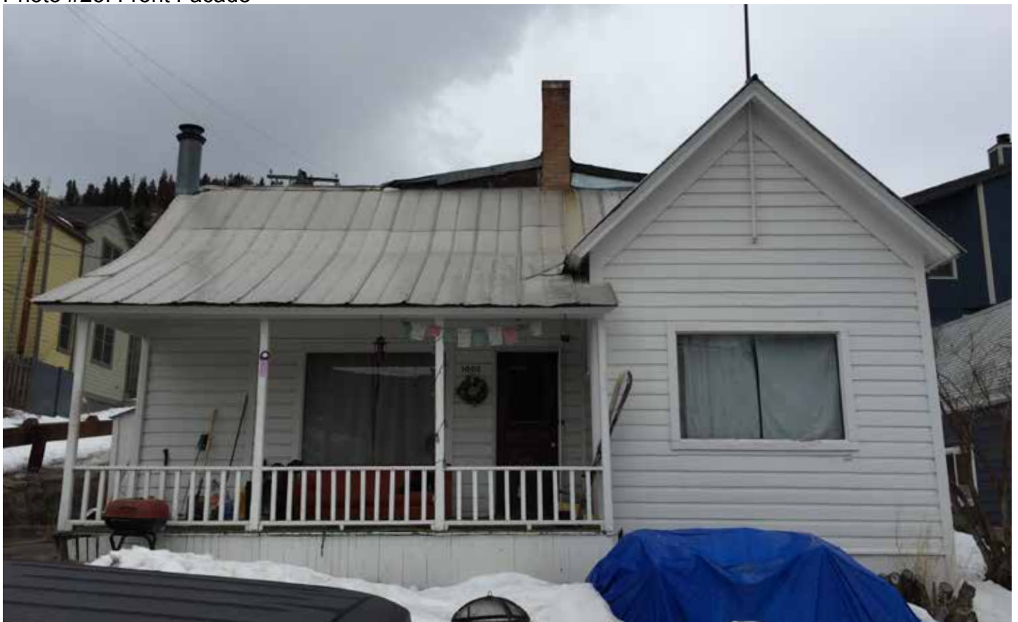
Photo #25: Front Facade
