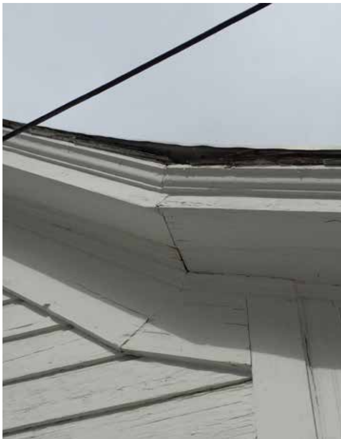
Photo #17: Detail of Roof Layers
