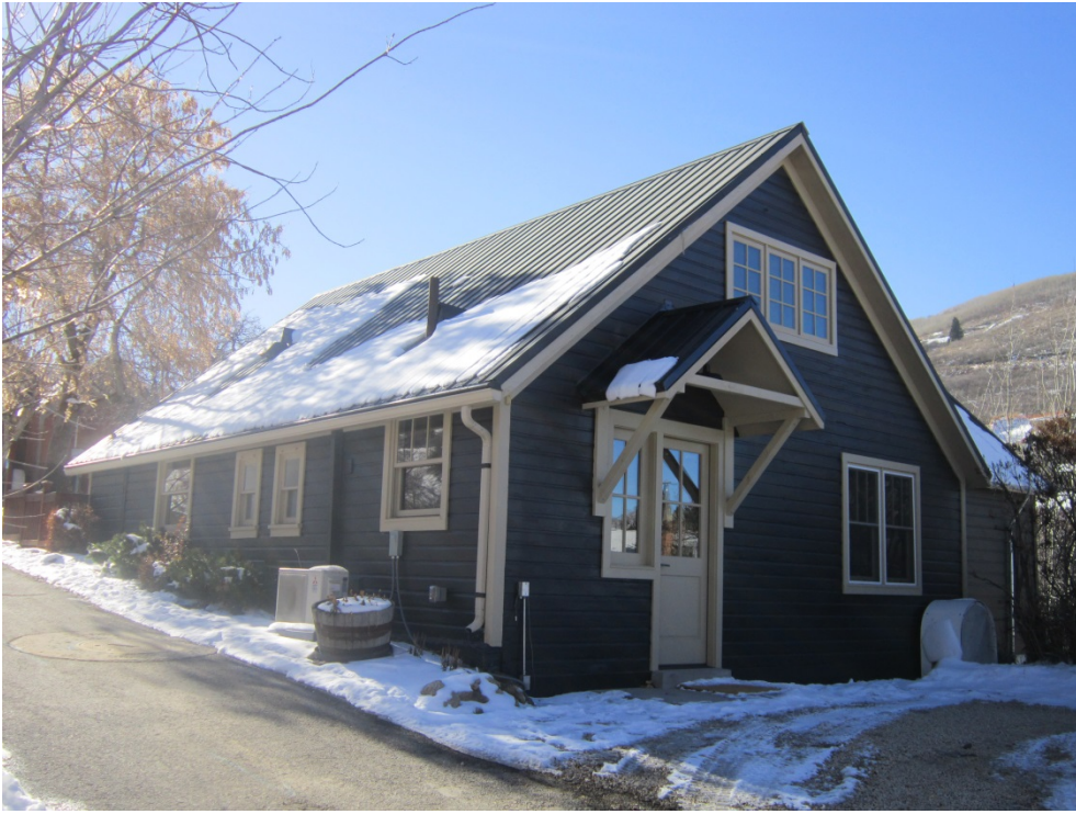
218 Sandridge Avenue. Northeast oblique. November 2013.
