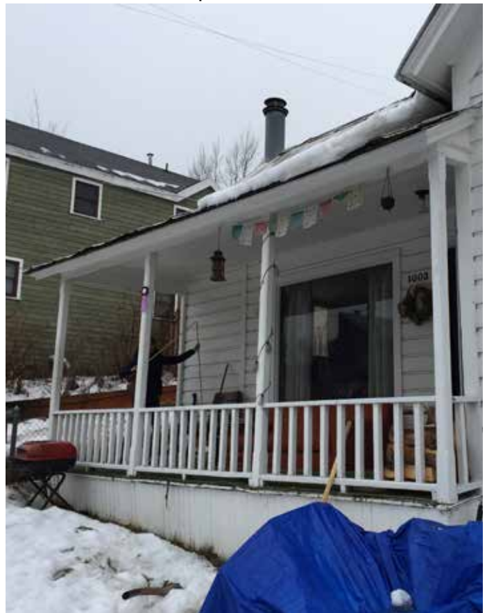
Photo #27: Close Up At Porch
