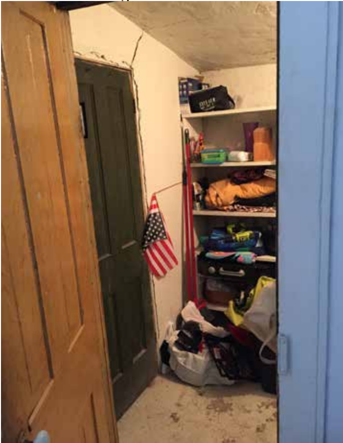
Photo #85: Storage Room
