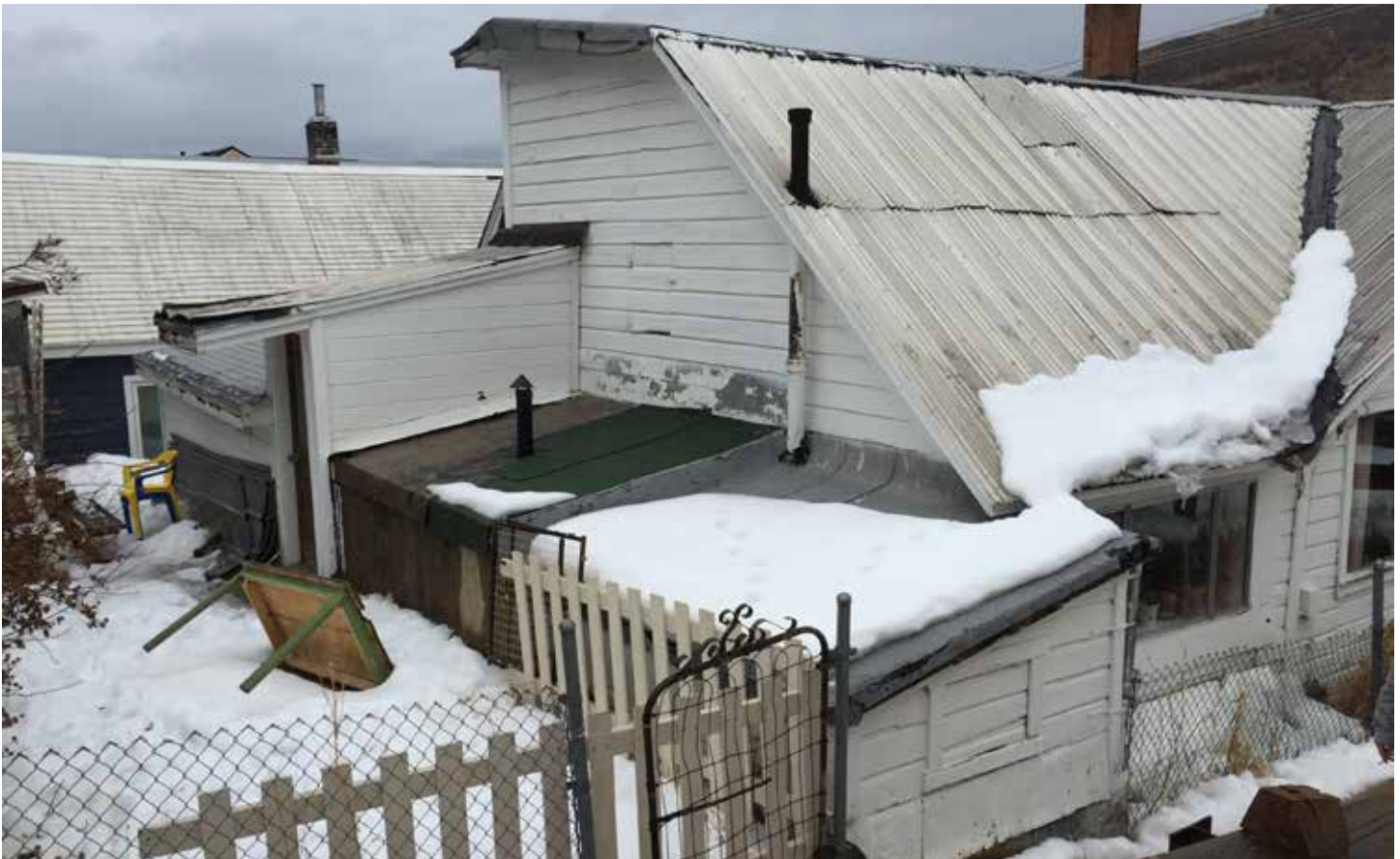
Photo #30: Rear Facade
