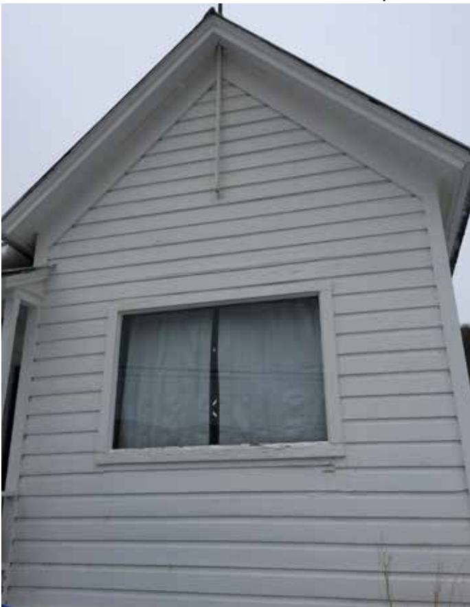
Photo #26: Gable Roofed Wall Close Up
