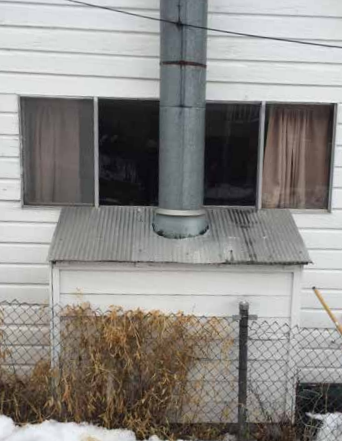
Photo #9: Low Shed Roof at Southern Side Yard
