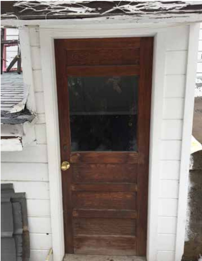
Photo #51: Door #2 From Exterior
