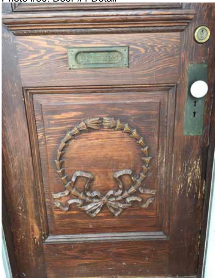
Photo #50: Door #1 Detail
