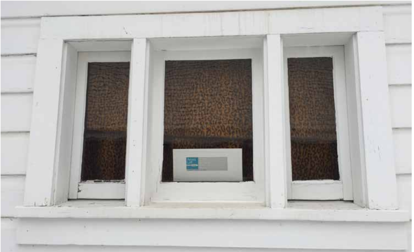
Photo #61: Window #9 From Exterior
