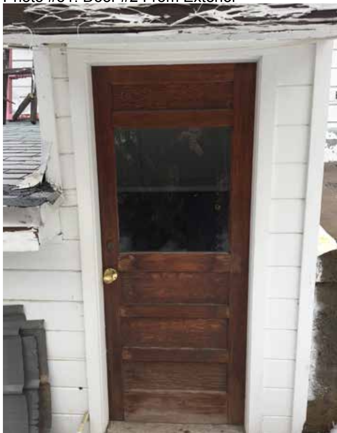
Photo #51: Door #2 From Exterior
