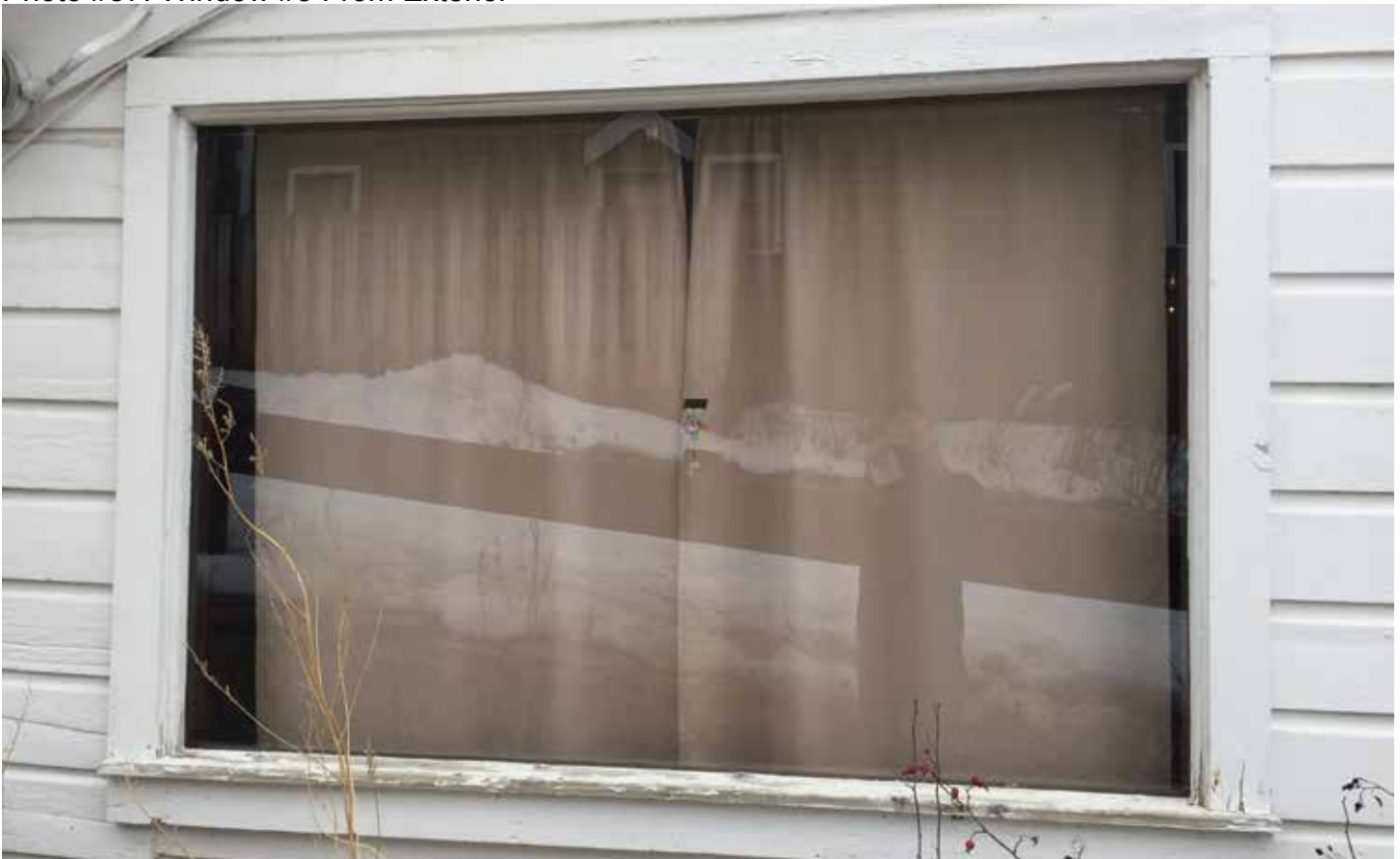
Photo #57: Window #5 From Exterior
