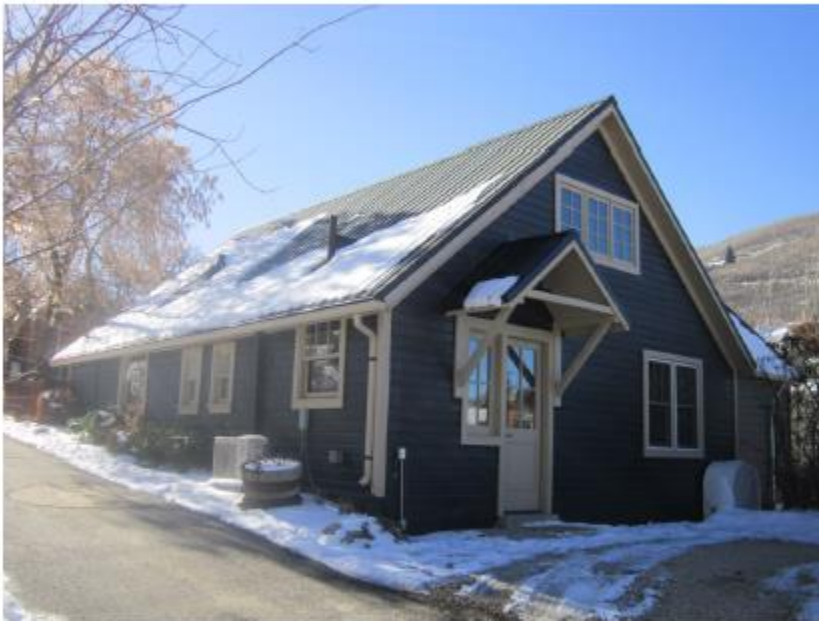
218 Sandridge Avenue. Northeast oblique. November 2013.
