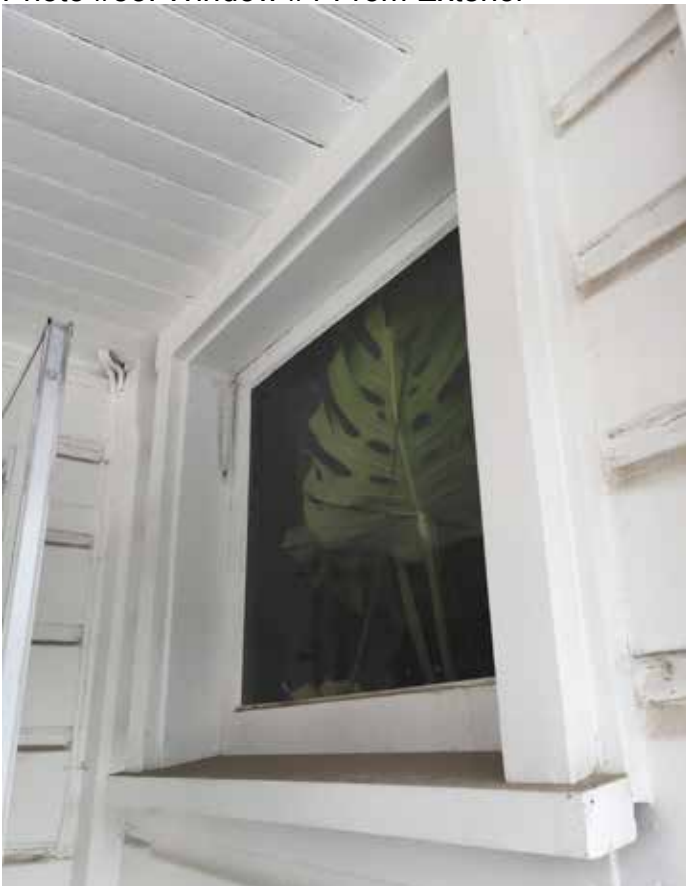
Photo #53: Window #1 From Exterior
