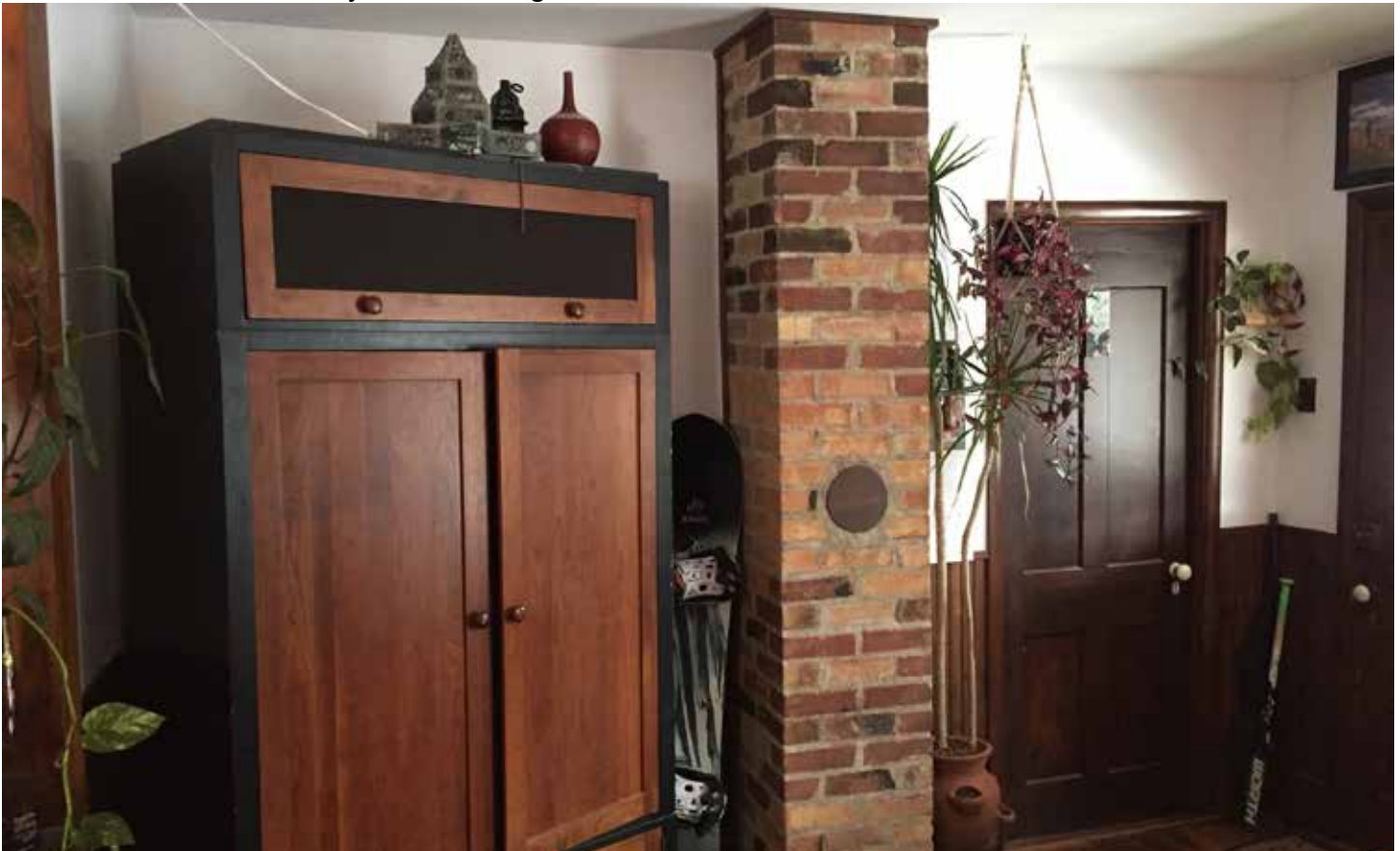
Photo #21: Front Chimney Within Living Room
