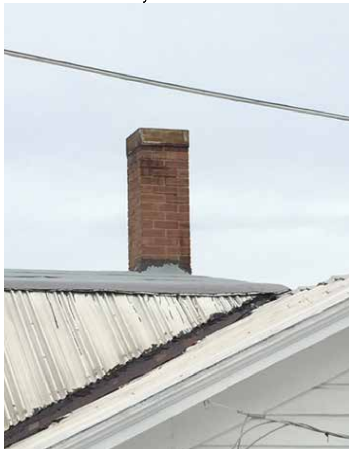
Photo #20: Chimney From South
