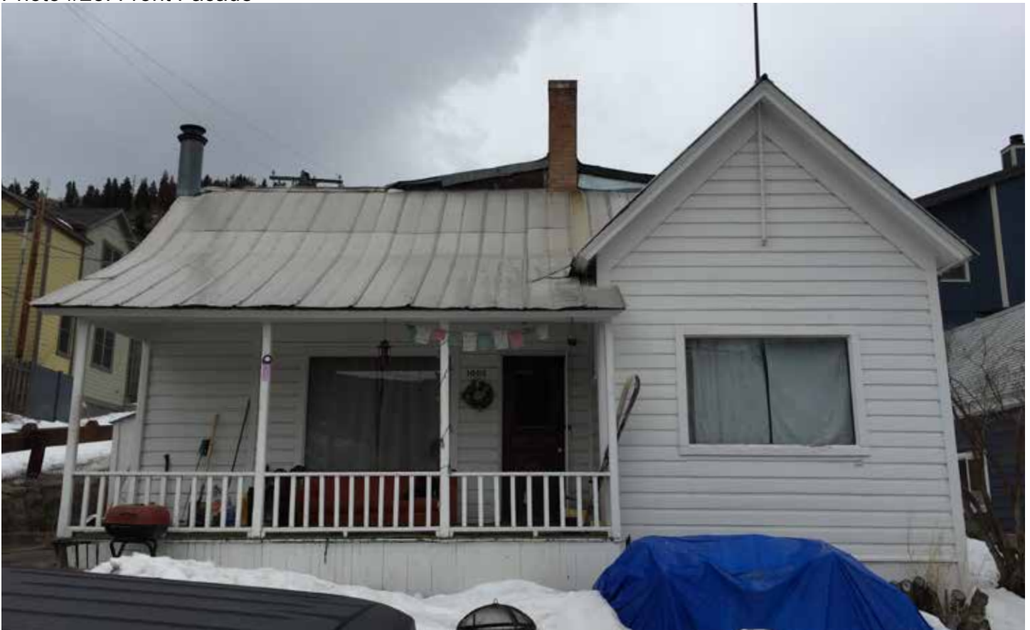
Photo #25: Front Facade
