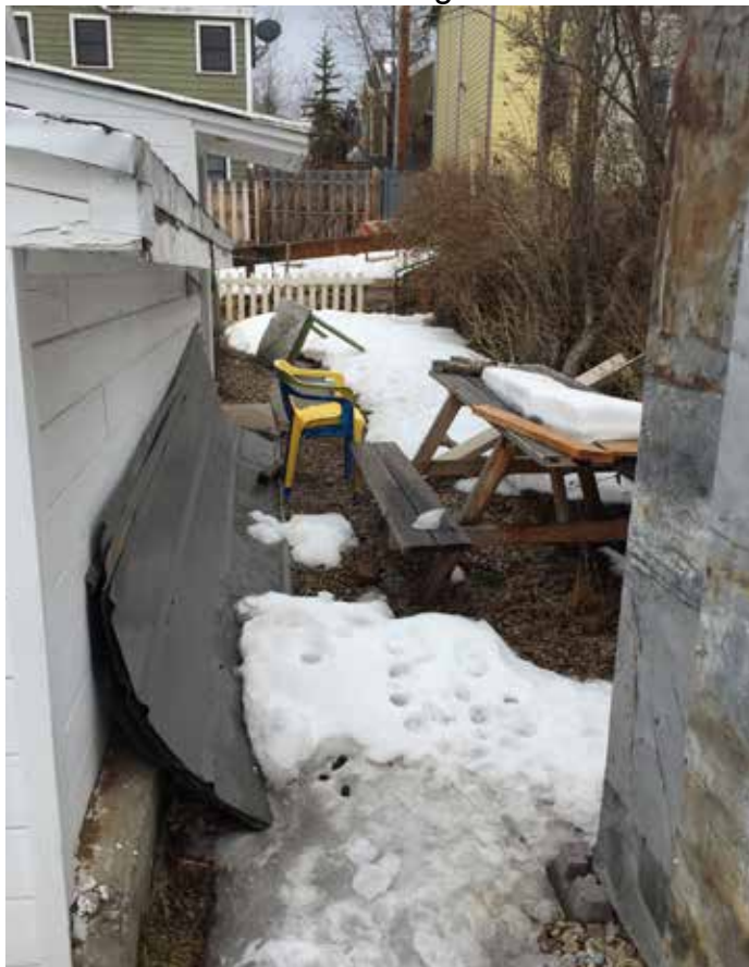
Photo #6: Rear Yard Grading
