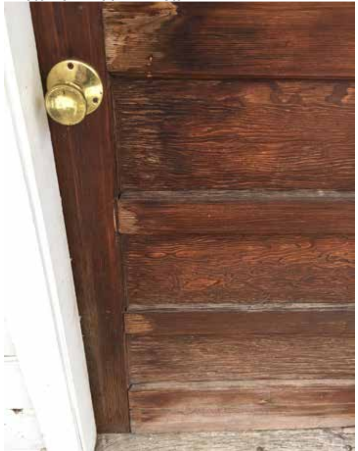
Photo #52: Door #2 Detail
