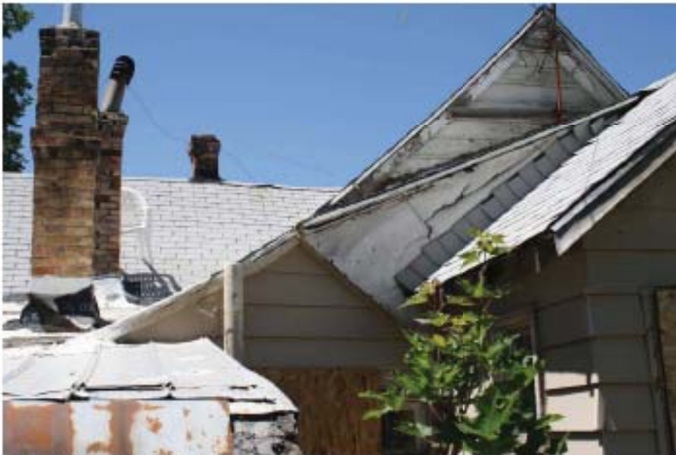
7. Toilet plumbing vent.
