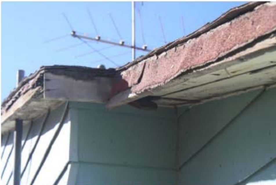
Transition from 6" overhang to 10" overhang
