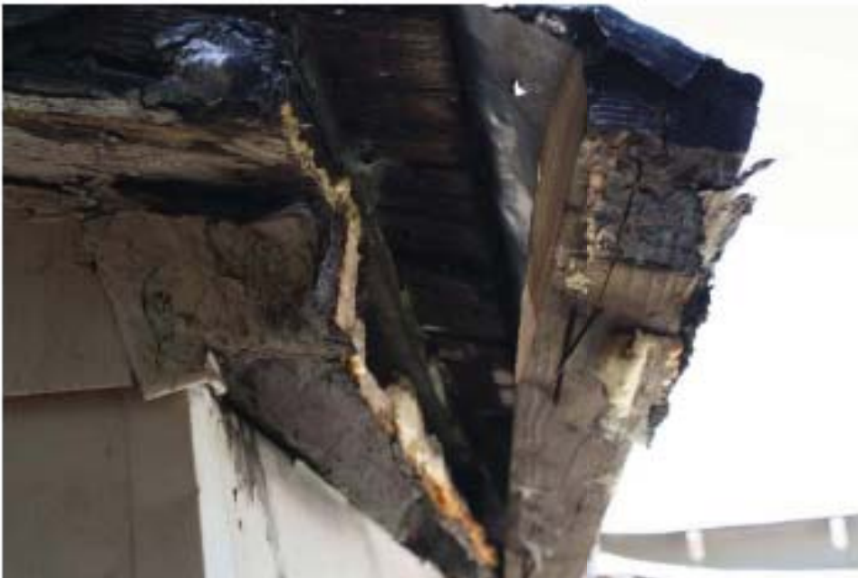
7. Fascia at southeast corner
