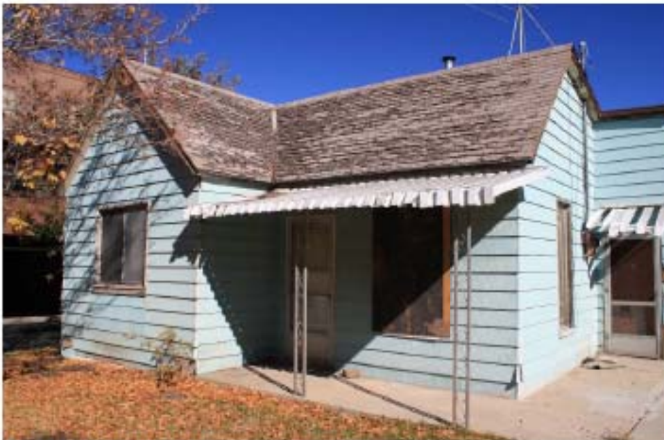
West front porch-2010
