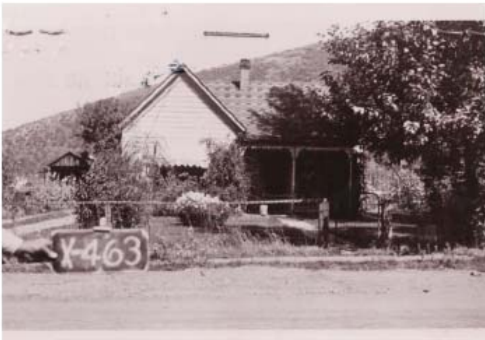
Historic front porch structure on 1450 Park Ave.
