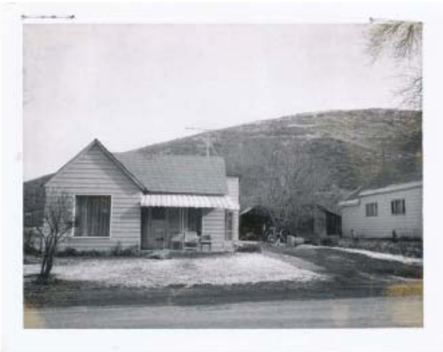
West front porch-1958
