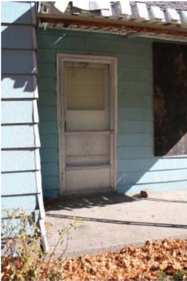
Concrete slab porch floor
