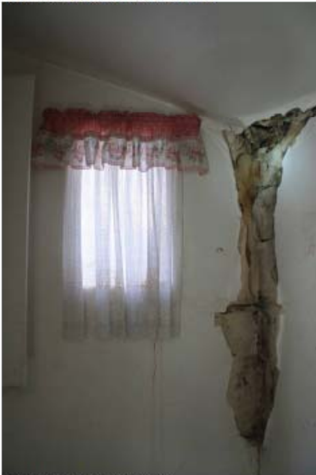
Interior northwest window
