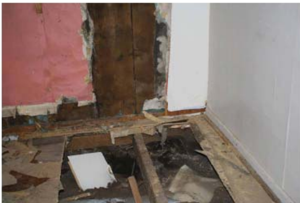
1. 1X12 wall construction. 2 1/8"X6" floor joist.
