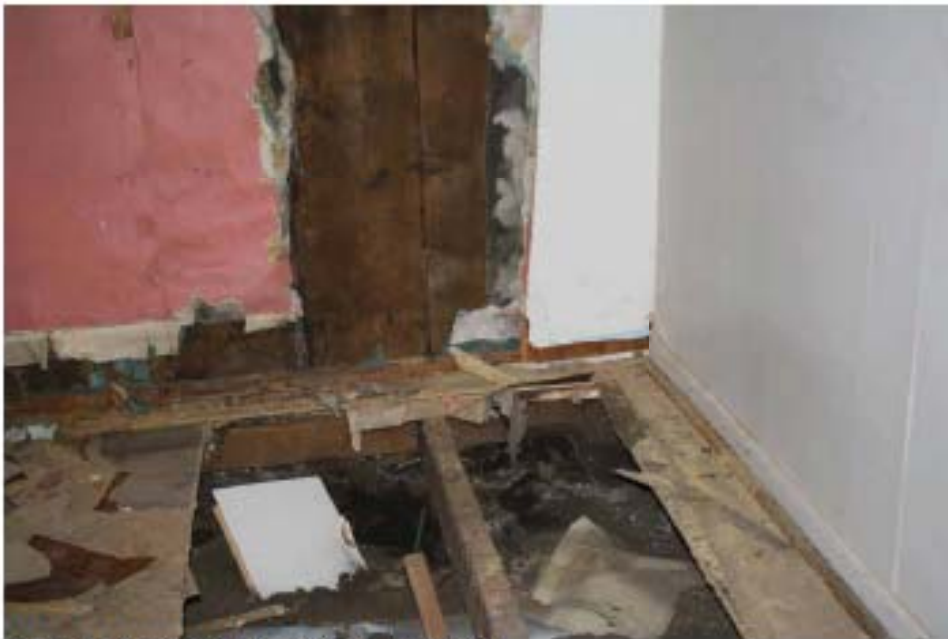
1.Look at interior excavation north wall
