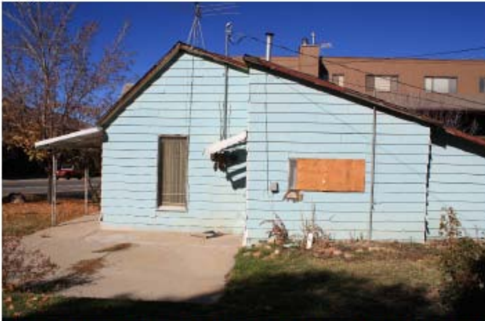
South windows-southwest 2'-7"W X 5'-8"H fixed 24"off slab. Center kitchen window 4'-11"W X 2'-0"H aluminum slider 3'-7" off ground. 2" historic wood casing
