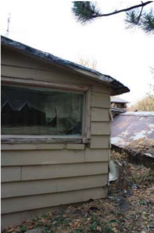
5. Southeast corner mechanical room
