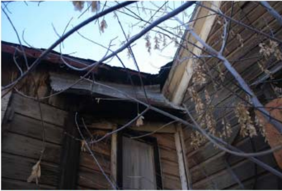
Corner- original 4'-0" shed structure
