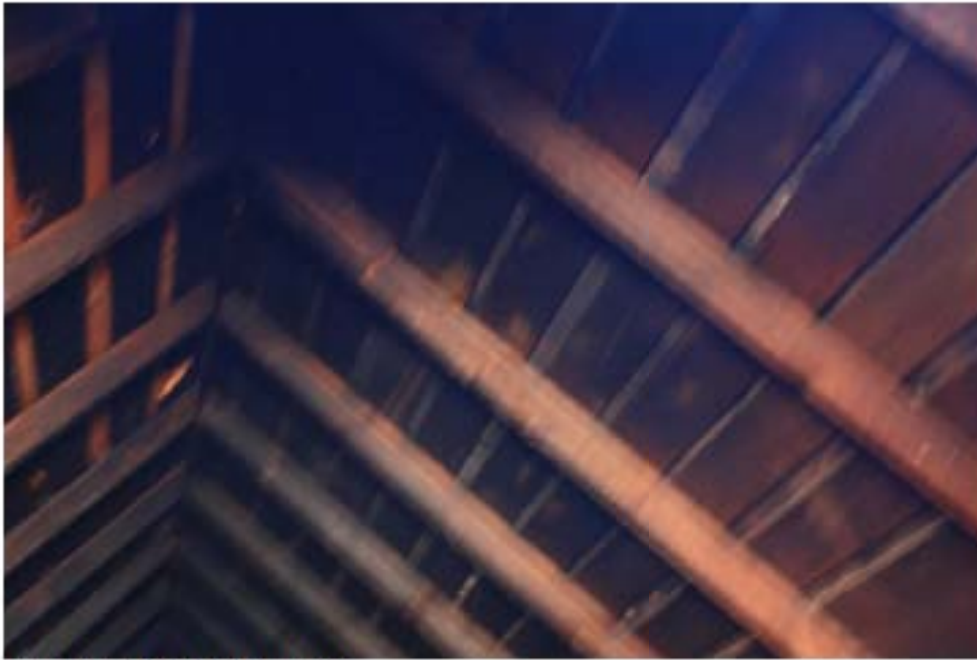
East-west gable framing
