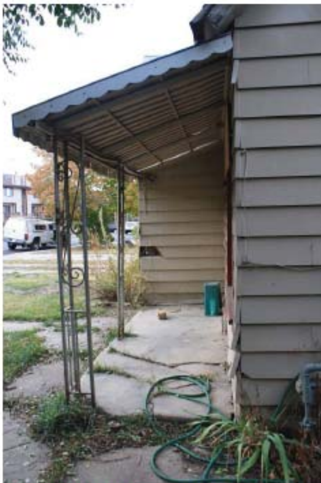
1.Original porch intersection-southwest corner
