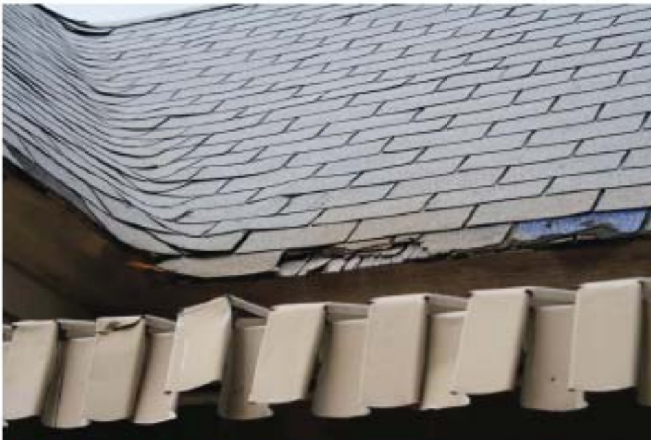
1.Original wood shingle
