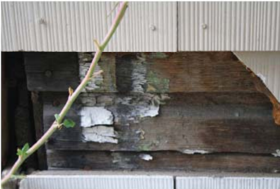
2. Siding detail northwest corner
