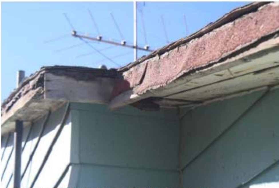
Soffit and fascia southeast corner kitchen/bathroom
