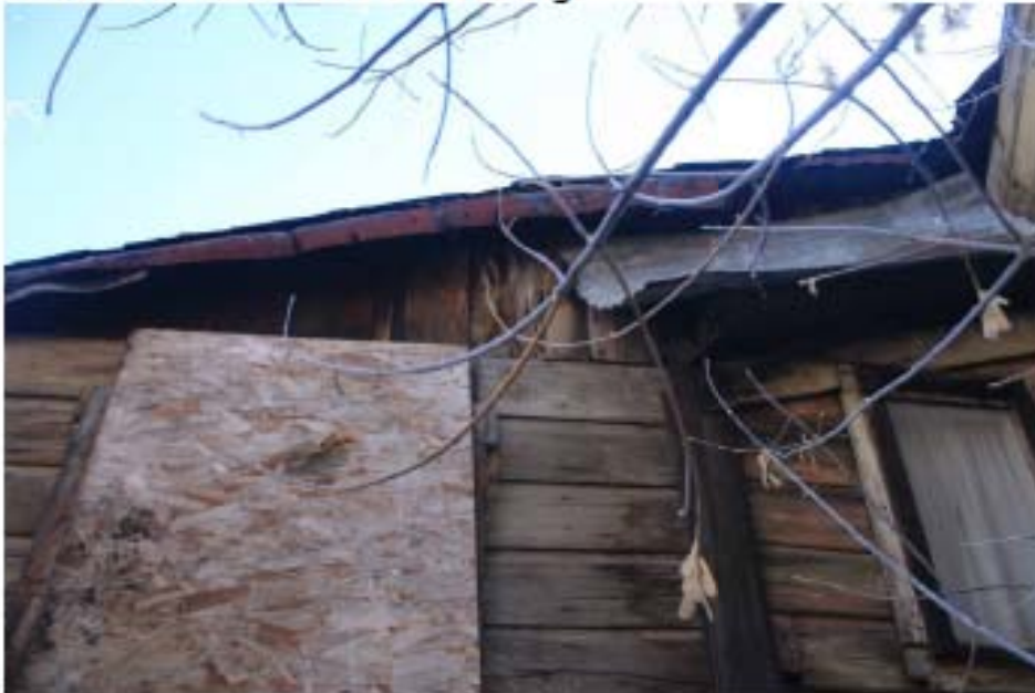
East bathroom window-modified casing
