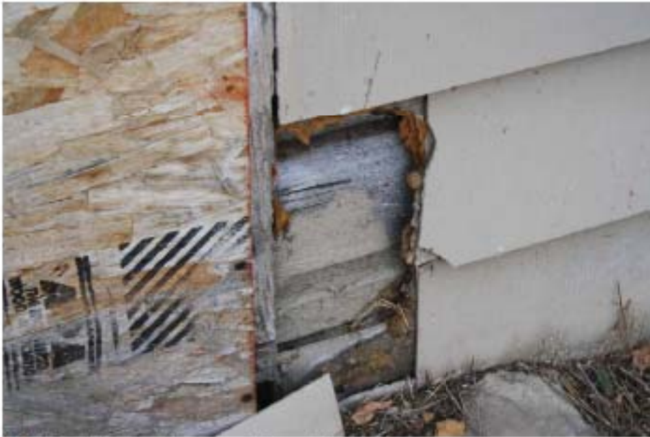
6. Siding detail-northwest gable north elevation
