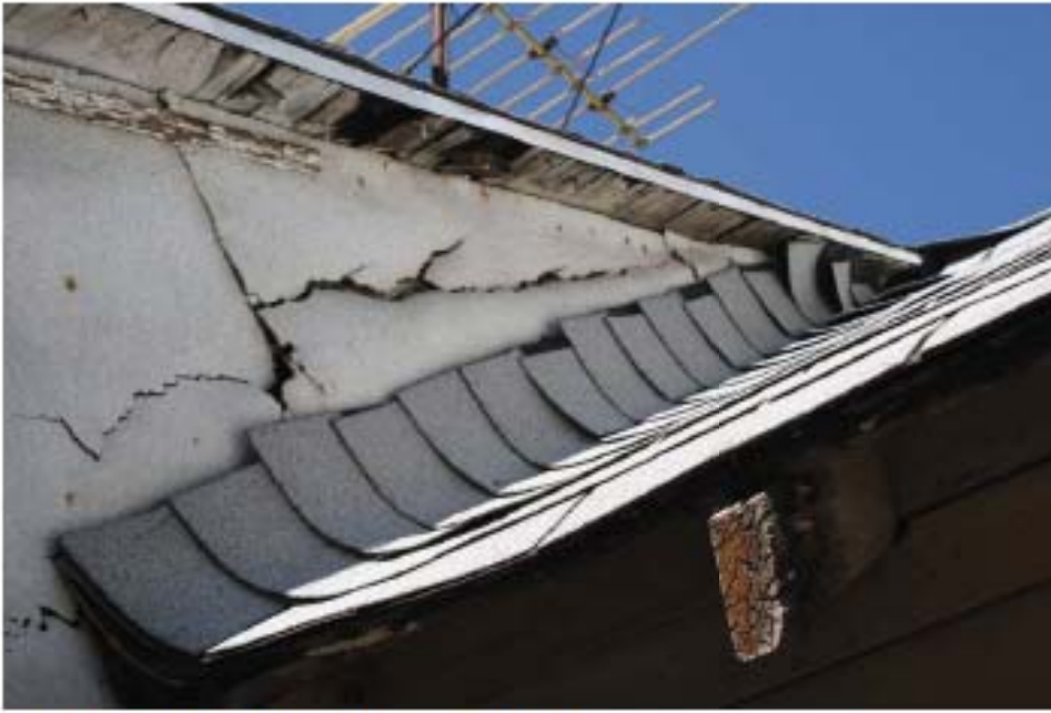
6. East elevation overbuild at bathroom
