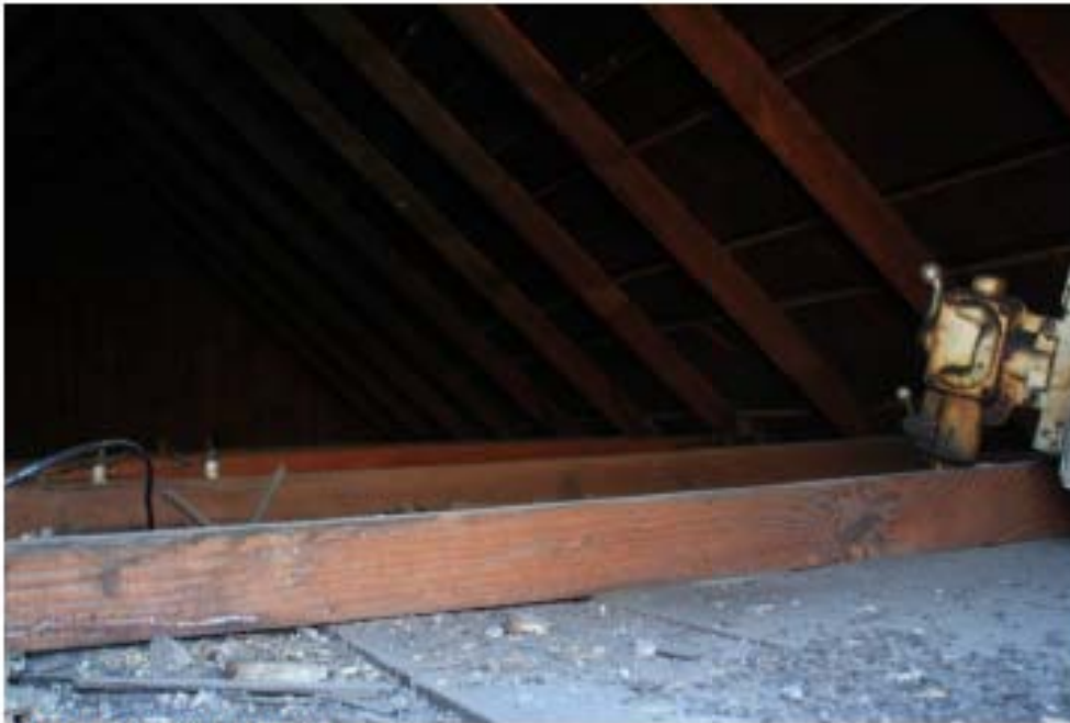
Roof and ceiling framing
