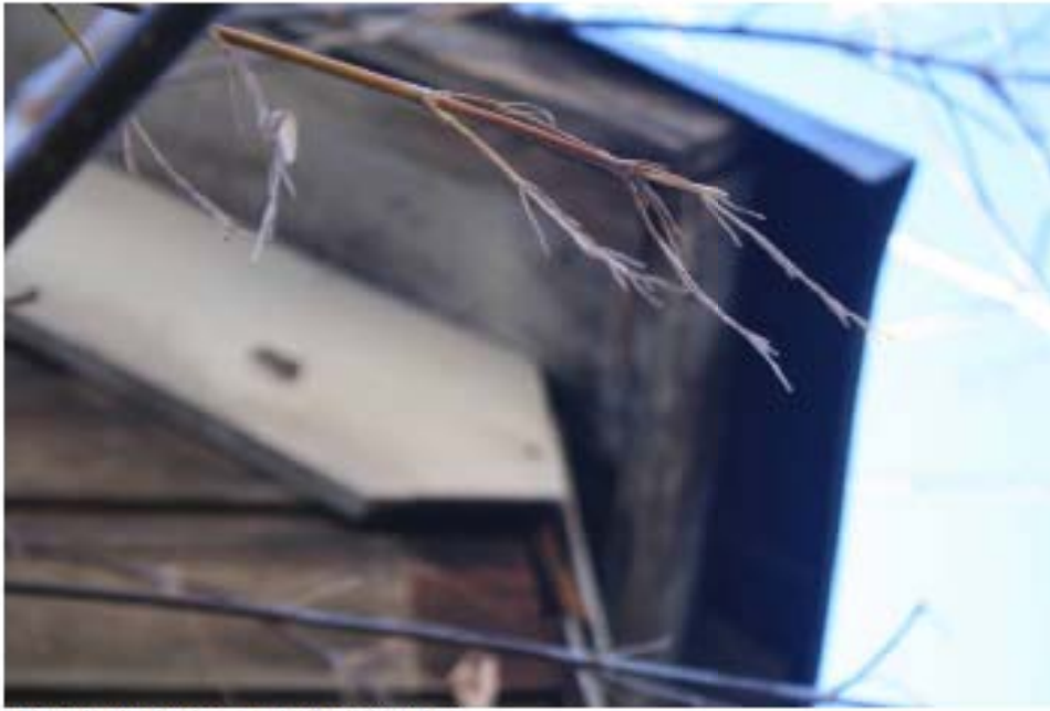
Wood 1X trim on east elevation
