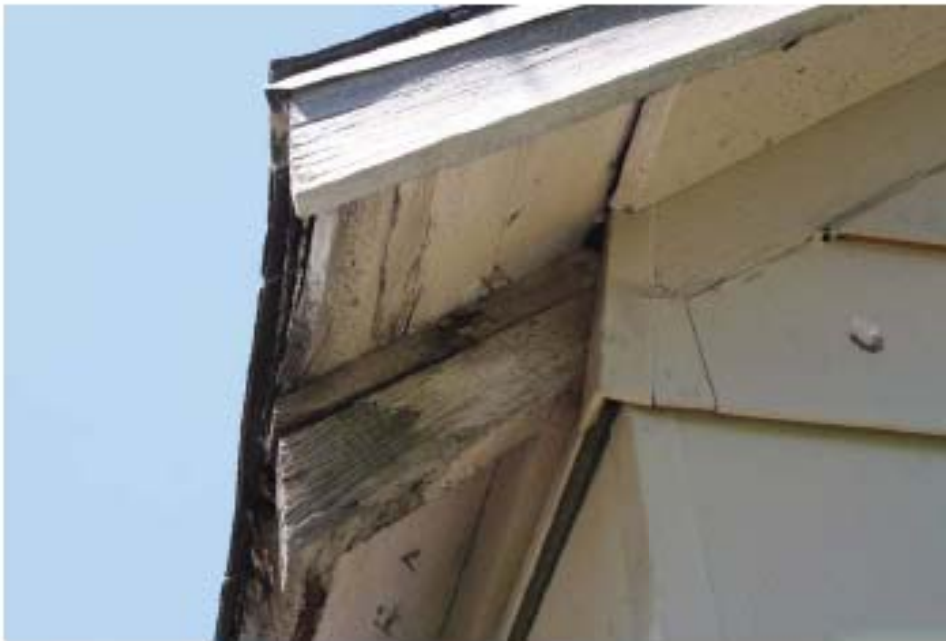
5.Soffit and fascia northwest corner
