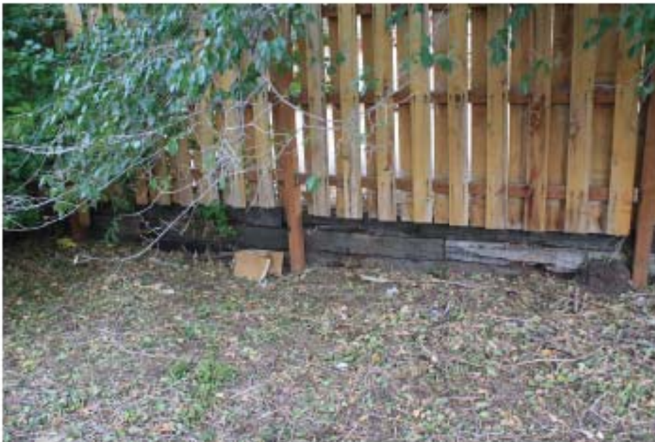
1.Railroad tie retaining wall
