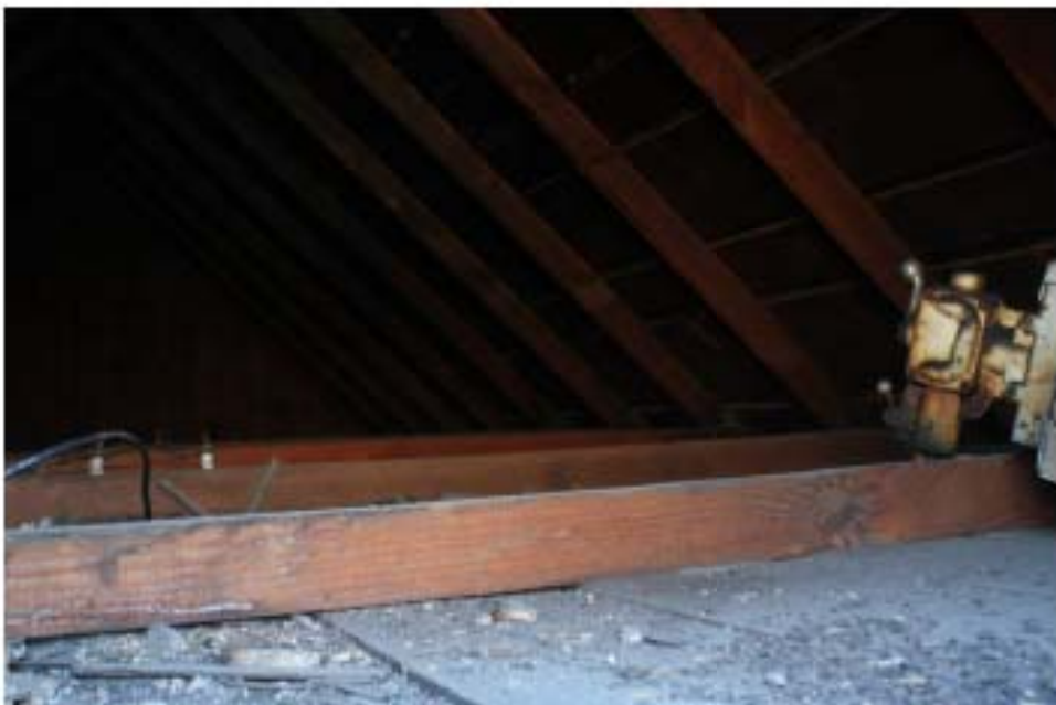
Knob and tube cloth wire-typical
