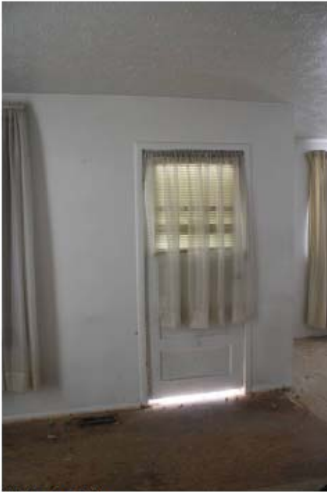
Interior front door
