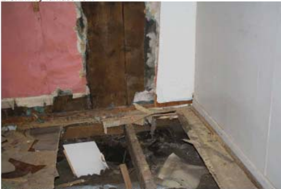
3. Duct work in foreground under floor joist
