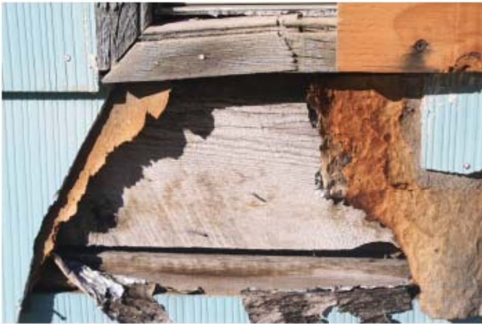
Typical 2" wood casing
