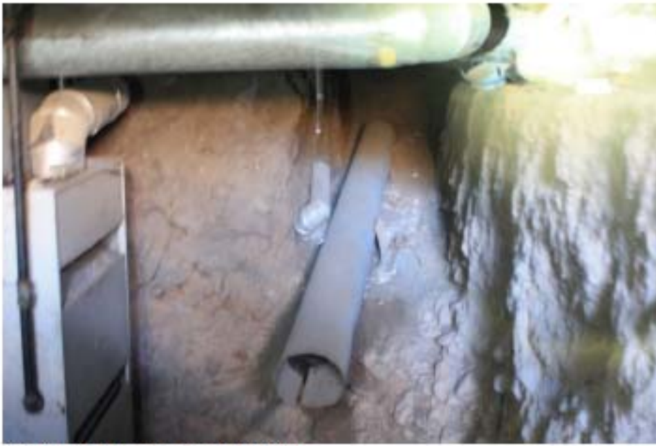
Duct work through excavated dirt
