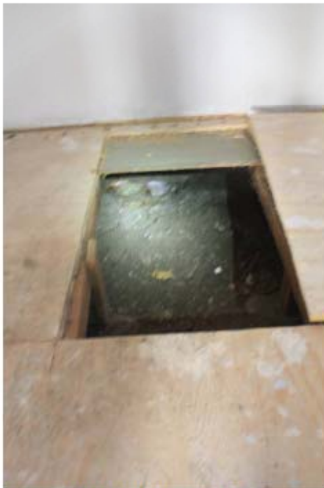
Foundation-floor joist on rubble stone
