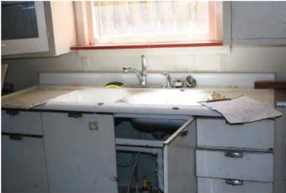
4. Metal kitchen sink and cabinet unit
