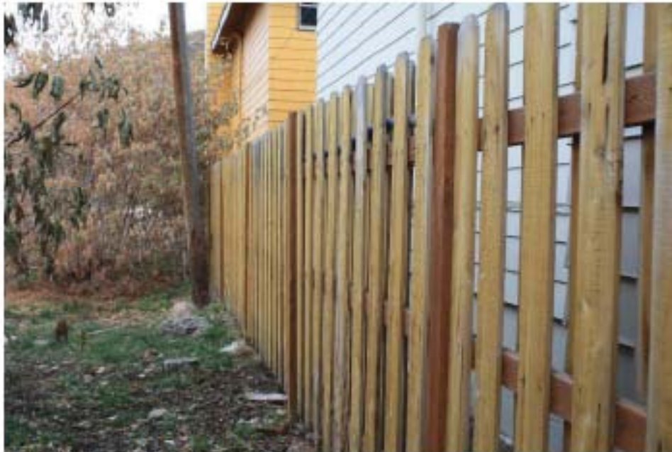
1.South property line wood fence
