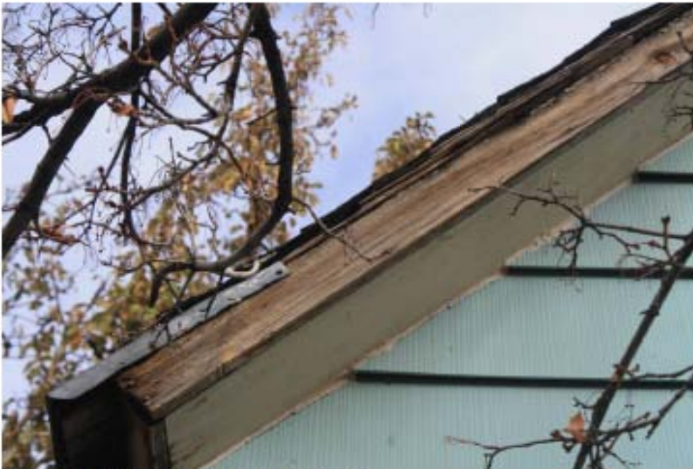
Soffit and fascia at northwest corner.
