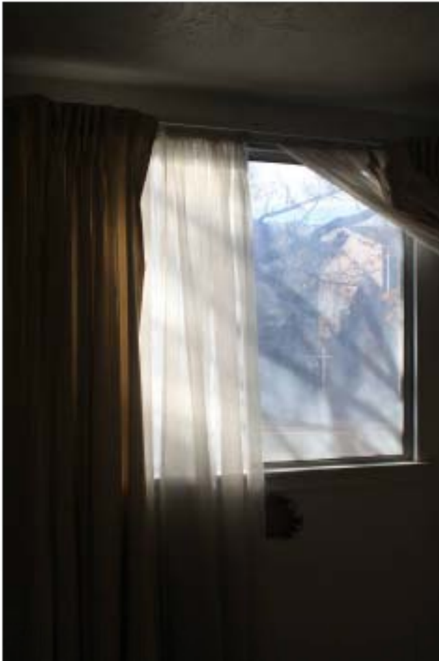
Front-west window interior-casing modified
