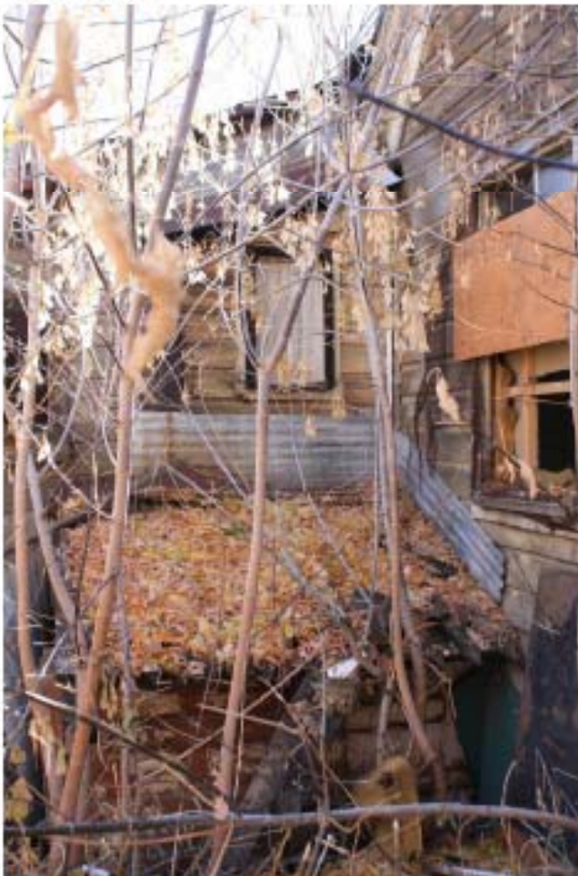
North elevation-shed access to mechanical
