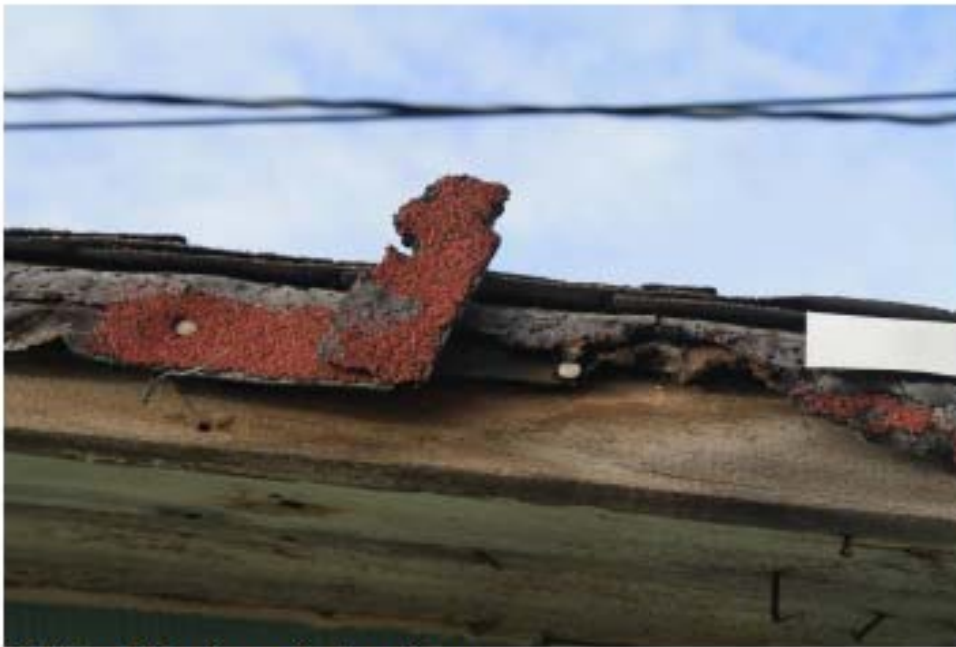
Soffit and fascia south elevation
