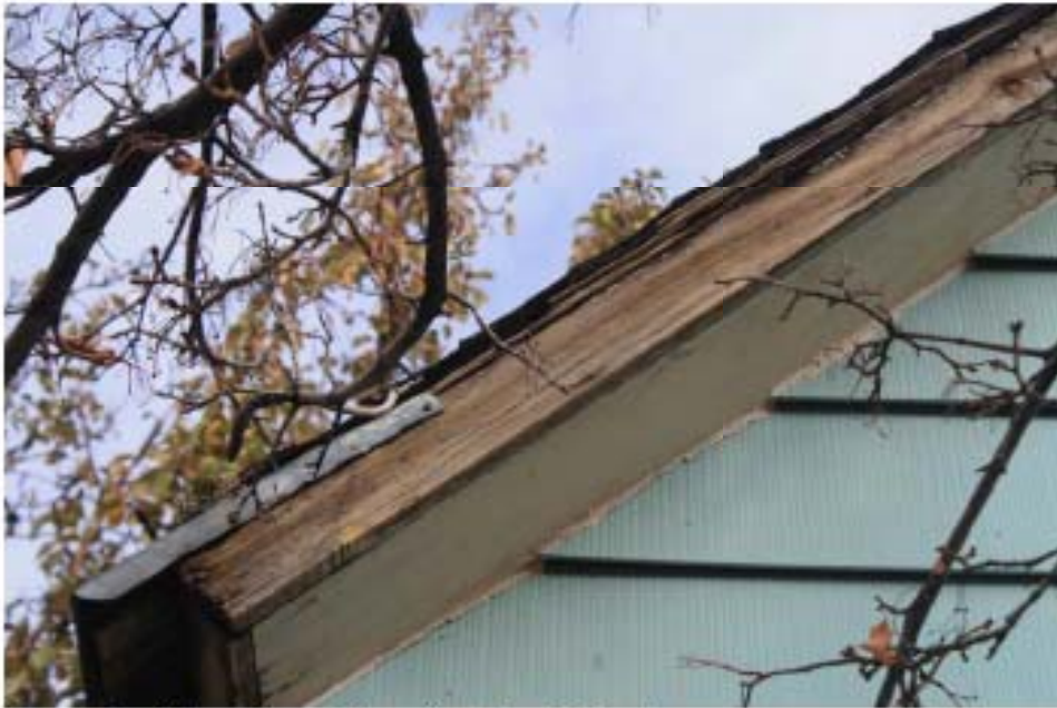
Typical soffit and fascia-functional and simple
