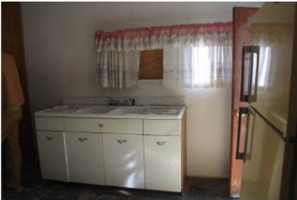
Kitchen sink south wall
