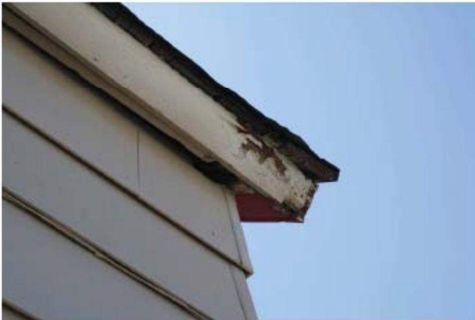
6.Fascia detail northeast corner
