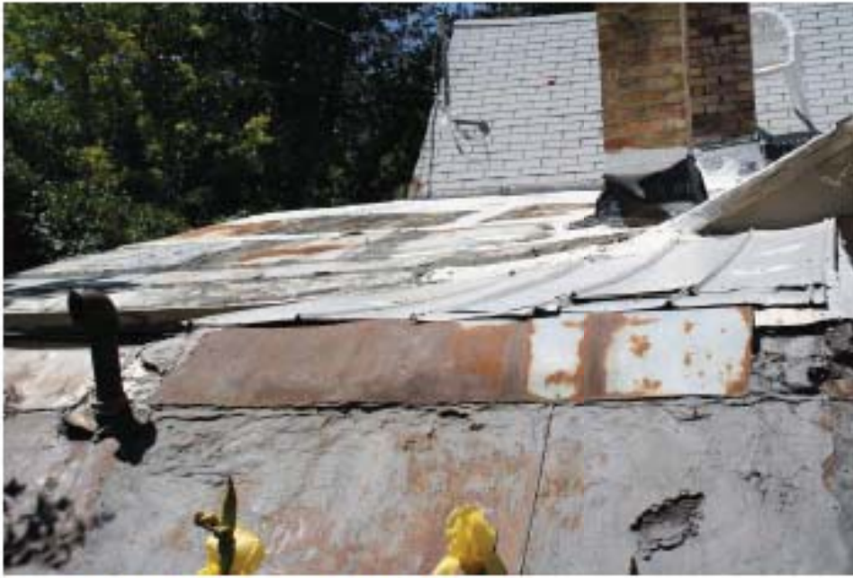
8. East elevation roof condition and chimneys
