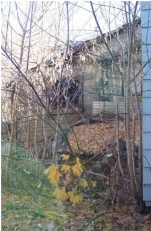
Topographical change at northeast corner
