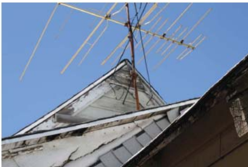
7. East elevation- original east/west gable
