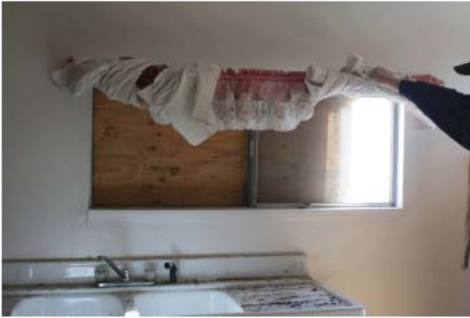
Interior kitchen window casing modified
