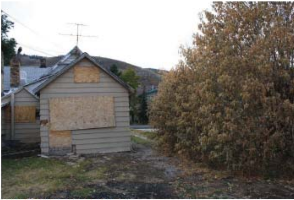
5. Northeast gable-north façade
