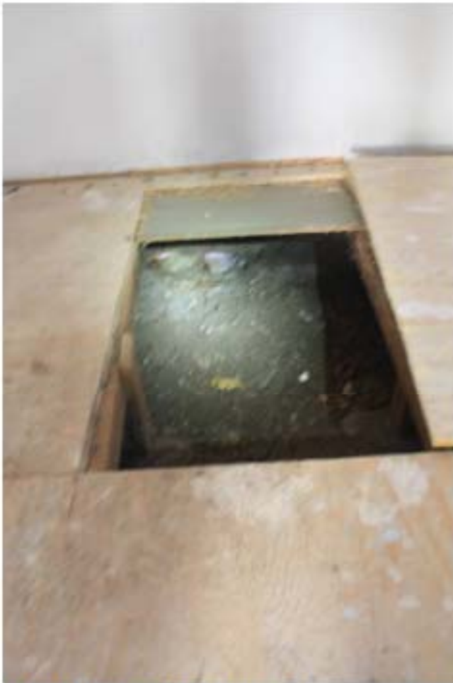
Dirt and rubble foundation-typical
