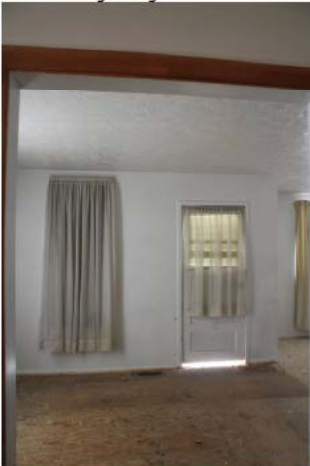
Ceiling lowered throughout house
