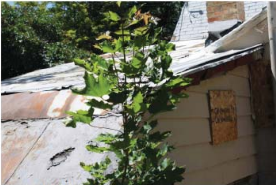
Window at stair to root cellar.
