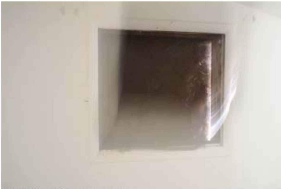
Northeast window-modified frame
