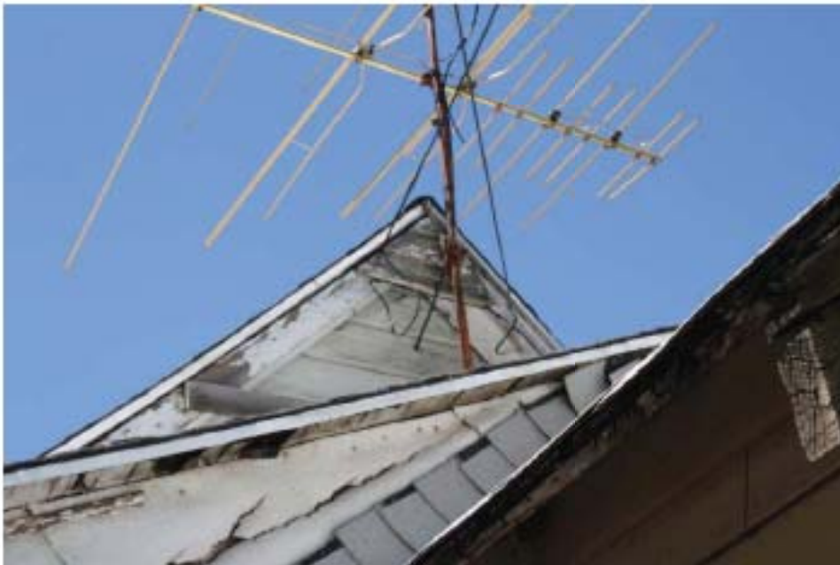
5.East elevation original gable
