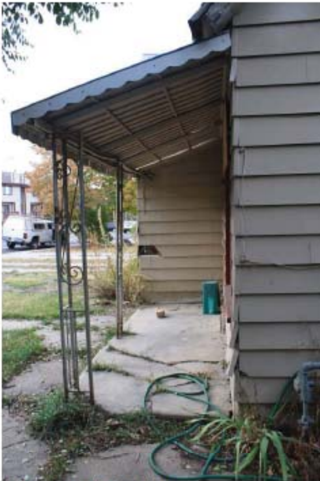
3. Porch- south elevation
