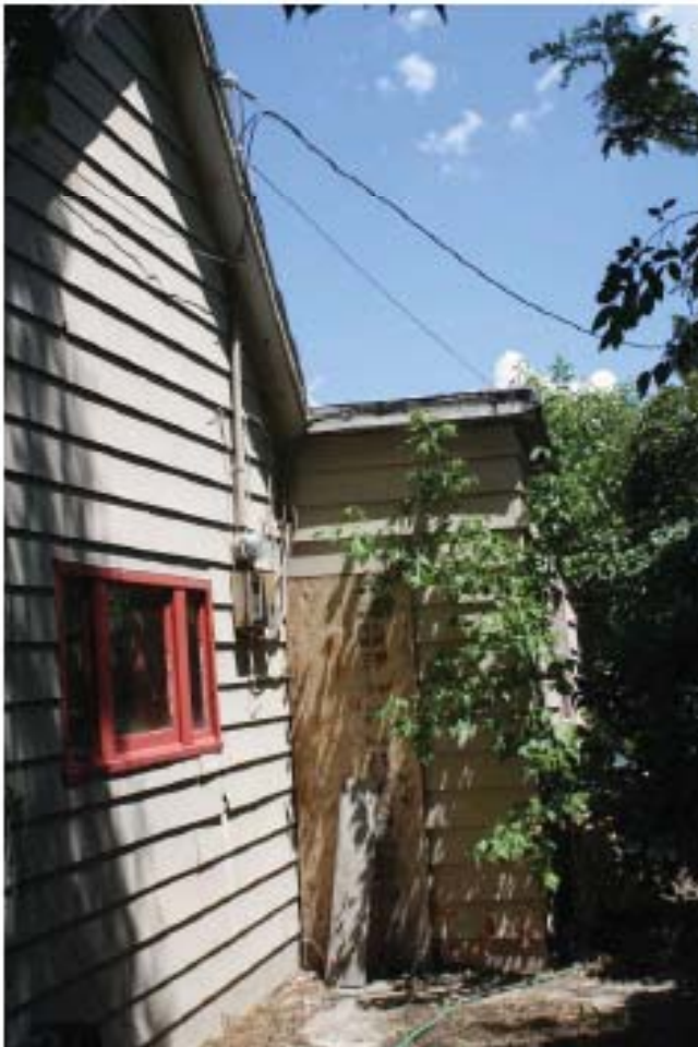
5. West kitchen door
