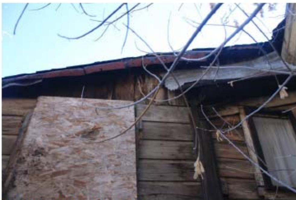
Intersection-sheds north elevation
