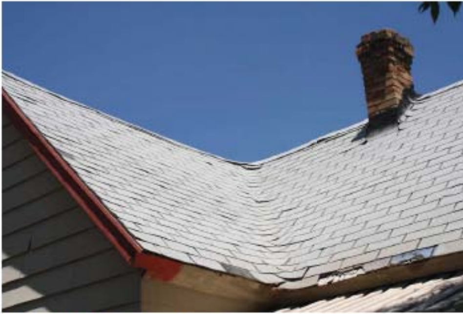
4.Original roof valley and chimney
