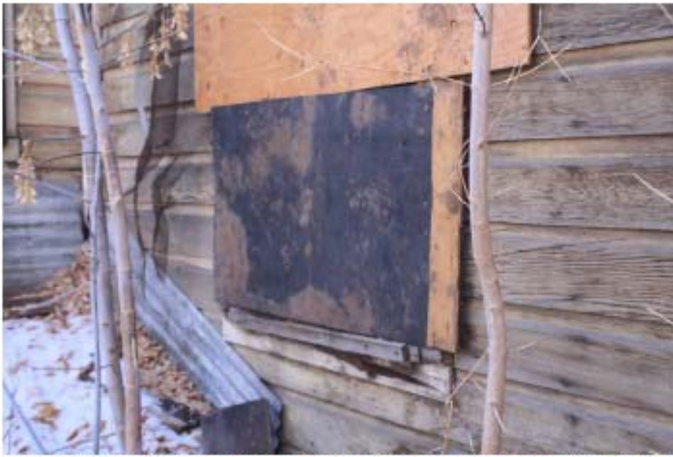
East bedroom window-existing aluminum slider 2'11"W X 2'-0"H and 6'-0" off floor Casing unknown. Historic window 2'-8"W X 5'-0"H 2'-5" off the floor- window style and casing unknown.
