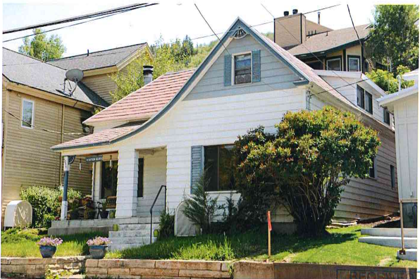
1055 Norfolk Avenue – Looking westerly
