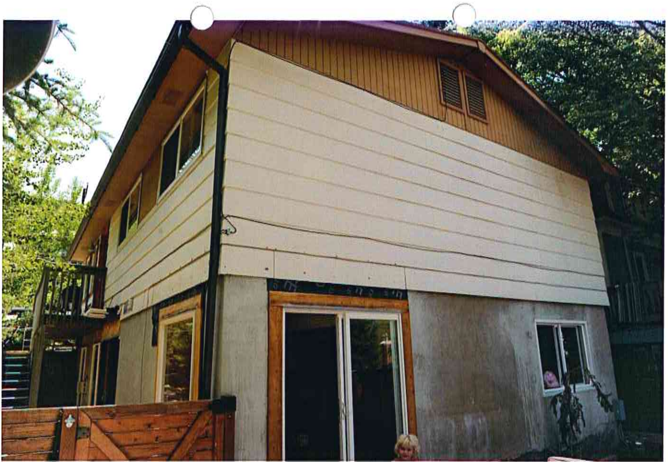
812 Norfolk Avenue – Looking westerly
